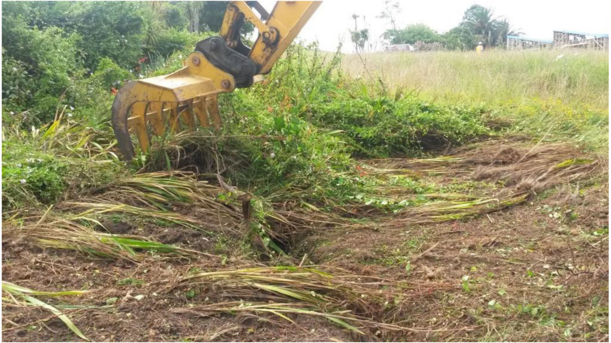
Figure 3 Excavator arm fitted with root raker
