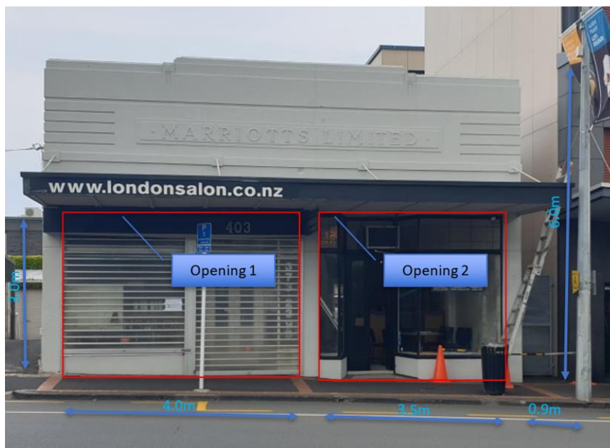
Figure 3. Existing frontage to be retained, access via openings
