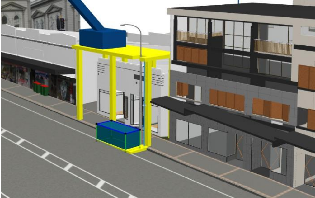
Figure 4. Platform mounted crane in front of the site entrance
