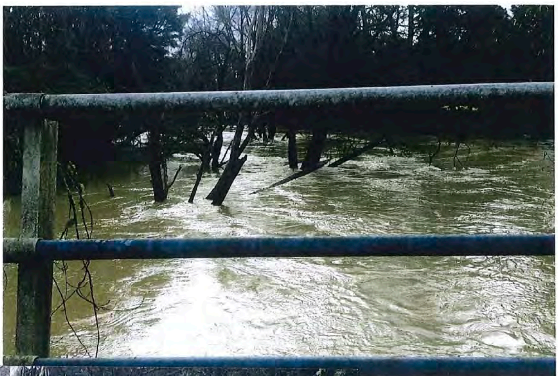
Leftover debris still coming loose 4 years later in 2016
