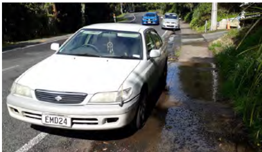
Figure 2: Footpath flush with road. Woodlands Park Road
