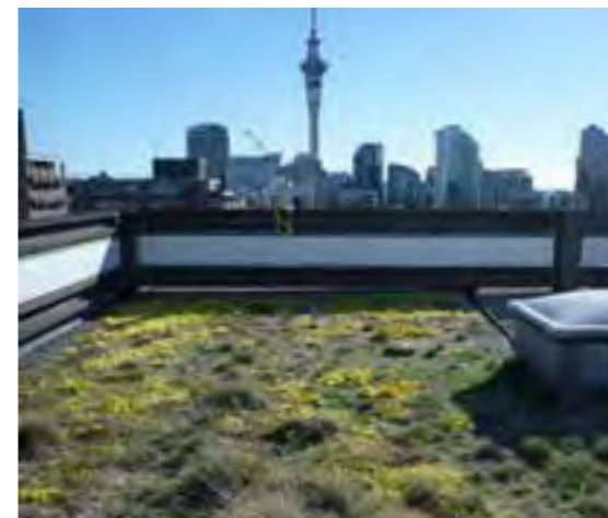
The University of Auckland green roof
