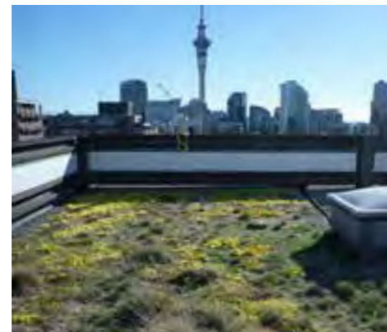
The University of Auckland green roof
