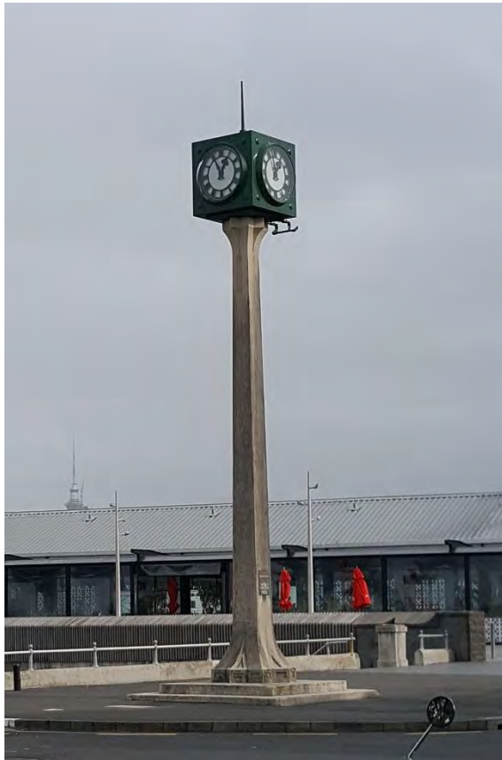
Figure 25: E. W. Alison Memorial Clock (Auckland Council; 24 June 2020)
