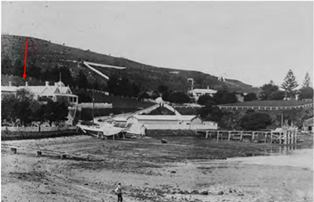
Figure 16. In this 1893 photograph the first phase of development of the submarine mining depot has been completed. A scoria seawall and reclamation have been built along the back of the bay to widen the access in front of the foreshore properties. The house at 62 King Edward Parade has been built and the earlier boatshed remains on the foreshore in front of the property. A tall tree (arrowed) visible in several photos of this end of the beach (see below) can be seen. Auckland Libraries Digital Reference Collection 4-2970
