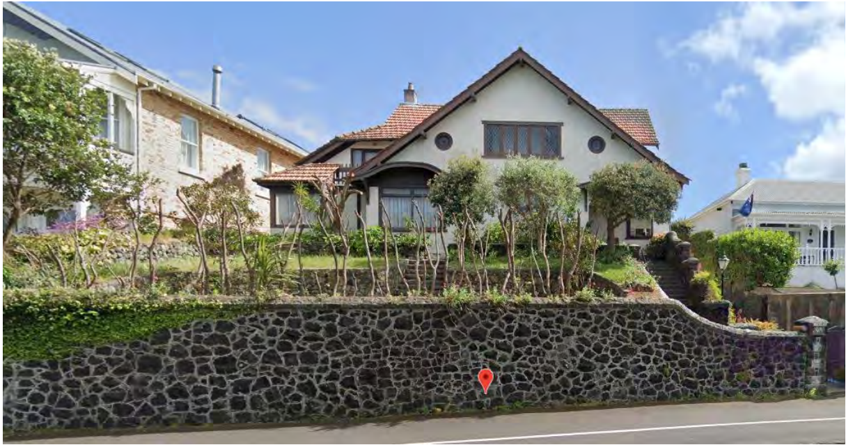
Figure 10. Rockcliff (ID 01107, Heritage NZ List 4518) at 6a King Edward Parade is built on the cut down rock outcrop that was formerly part of Magazine Rock. The stone walls, pillars and landscape features are likely made from the rock. Rockcliff is the subject of another A* review. Source: Google Street View.
