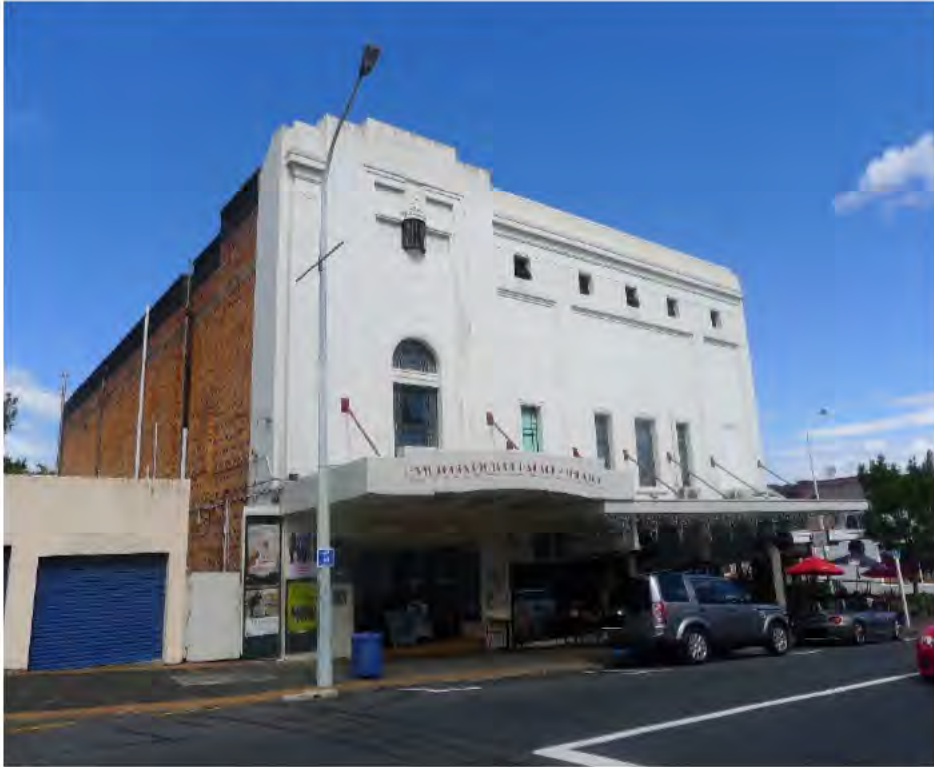
Figure 10: Victoria Theatre (Auckland Council 2013)
