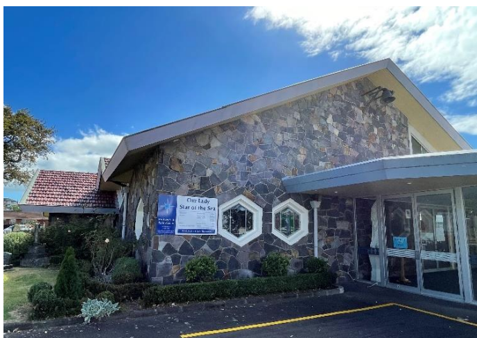
Figure 6: The southern elevation front entry on the western side to the church, showing the enclosed carport which is now a foyer entry. (Auckland Council, March 2022)
