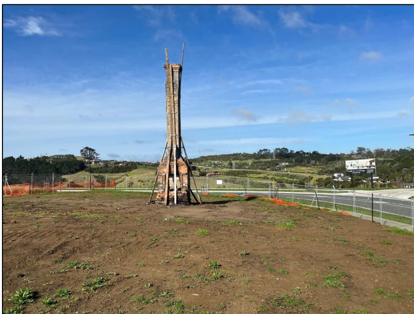
Figure 1. Remains of Major Bremner's Cottage following the fire and clearance of site (DPA Architects 31 May 2022).
