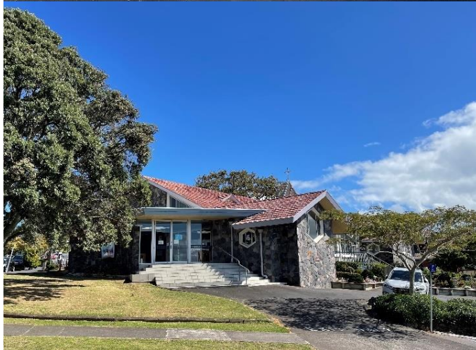
Figure 7: The southern elevation front entry on the eastern side to the church, showing the enclosed carport which is now a foyer entry. (Auckland Council, March 2022)
