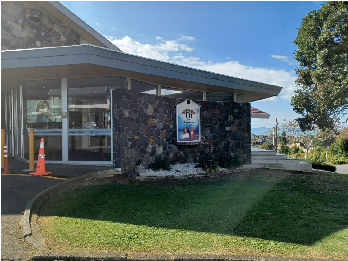
Figure 8: The original curved rock wall of the former carport, on the southern elevation. Clear views to the sea providing the setting for the naming of this church. (Auckland Council, May 2022)
