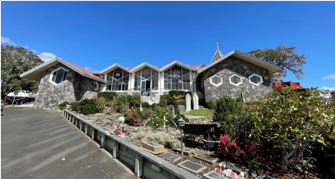
Figure 11: The eastern elevation, showing side entry and terrace. (Auckland Council, March 2022)
