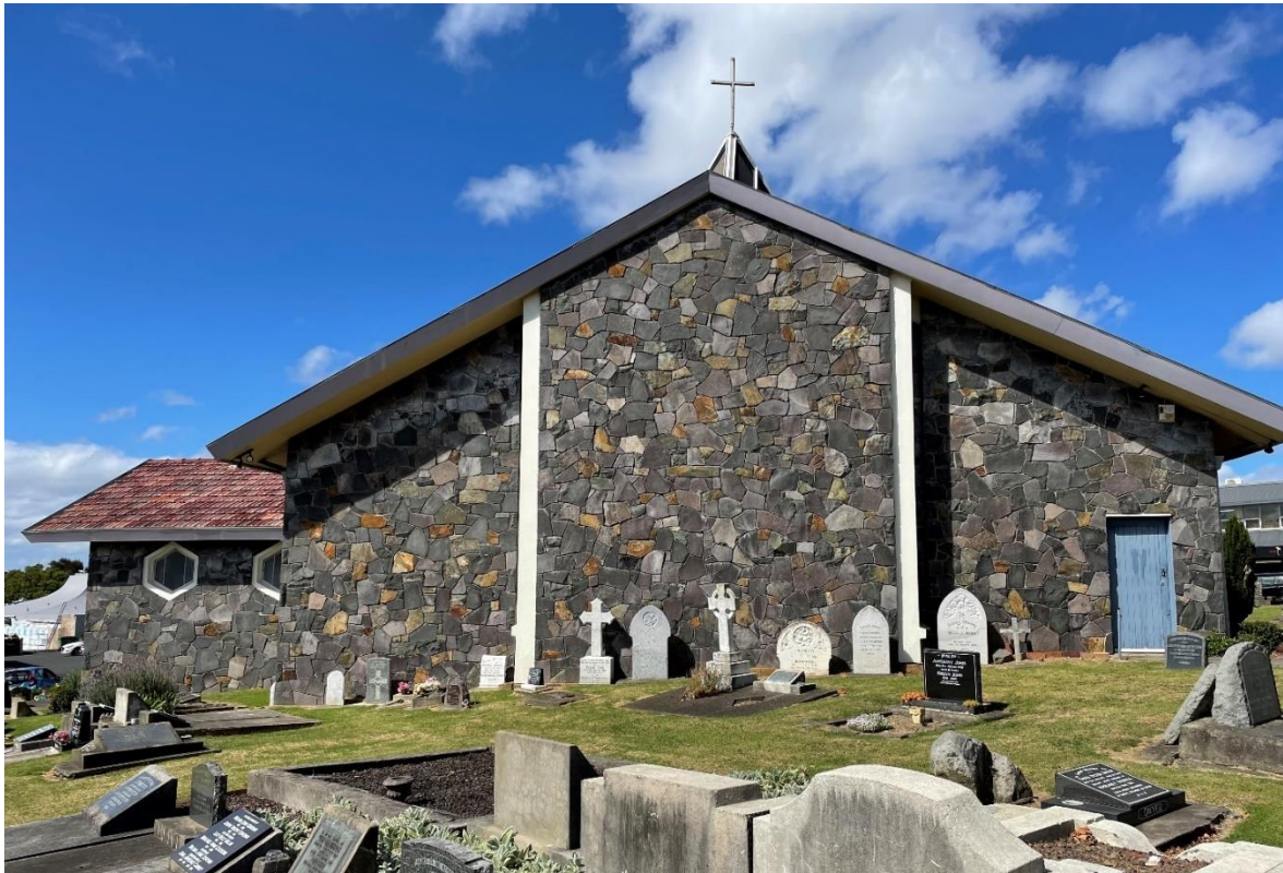
Figure 10: The northern elevation (Auckland Council, March 2022)
