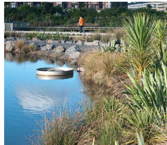
Example of Stormwater Pond Landscape Treatment
