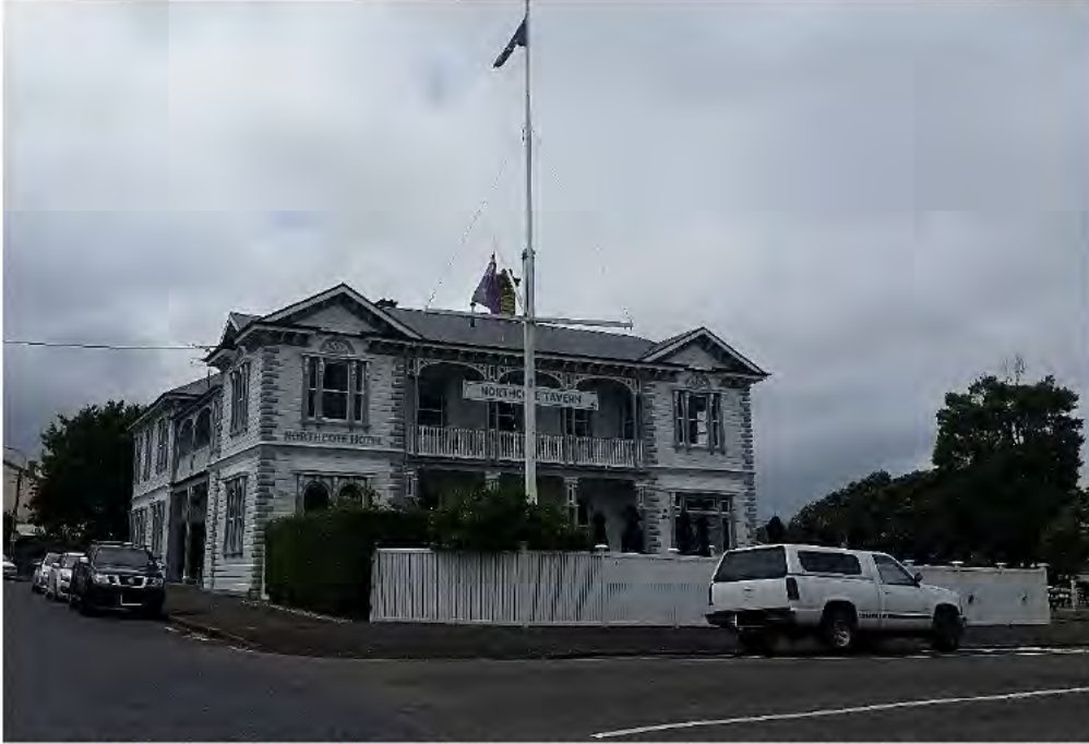
Figure 62: Northcote Hotel (former), 37 Queen Street, Northcote Point (Auckland Council, 28 October 2020).
