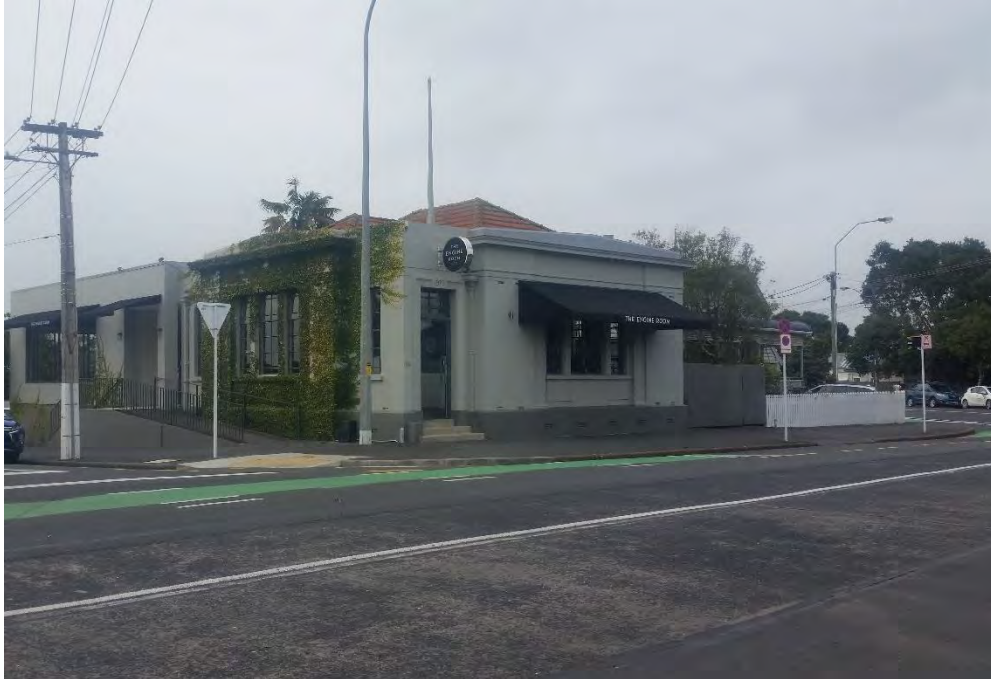
Figure 66: Northcote Post Office (former) (Auckland Council August 2020)
