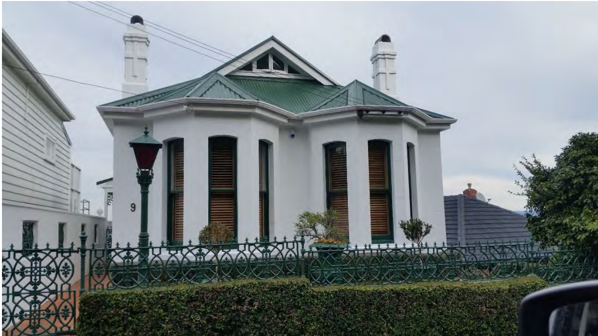
Figure 12. Gilderdale Thompson residence (Auckland Council, 23 May 2020)
