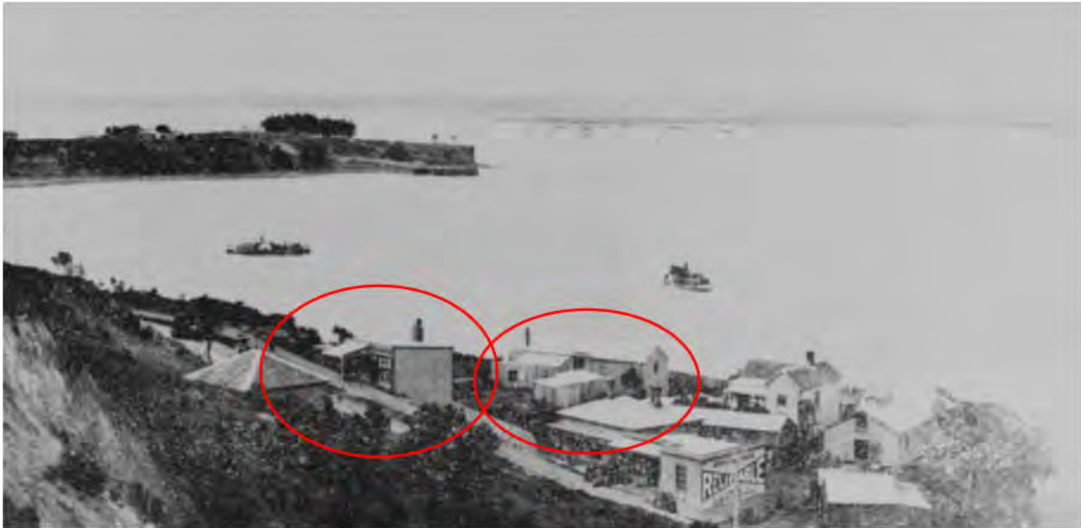
Figure 14. The land now known as 7 and part of 9 Hinemoa Street in a photograph taken before any houses were built on the Thompson land. The shop that Thompson owned is shown in the circle to the left. The sheds at the rear shown in the circle to the right are possibly the canning factory set up by William Thompson. (Auckland Libraries Heritage Collections B0518).
