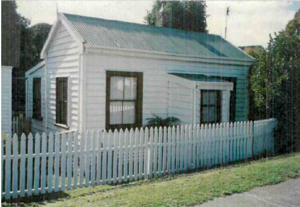
Figure 3. This is an image taken from Dinah Holman's report dated May 1994, demonstrating a more original version of the house. The sizeable addition has compromised the readability of the early cottage. (NSCC Site Pack).
