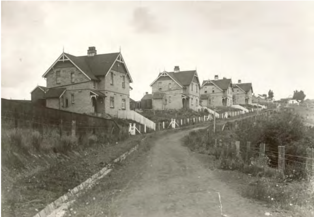
Figure 8. The Chelsea Estate Refinery Cottages in 1910 soon after they were built. (Auckland Libraries Heritage Collections B0063).
