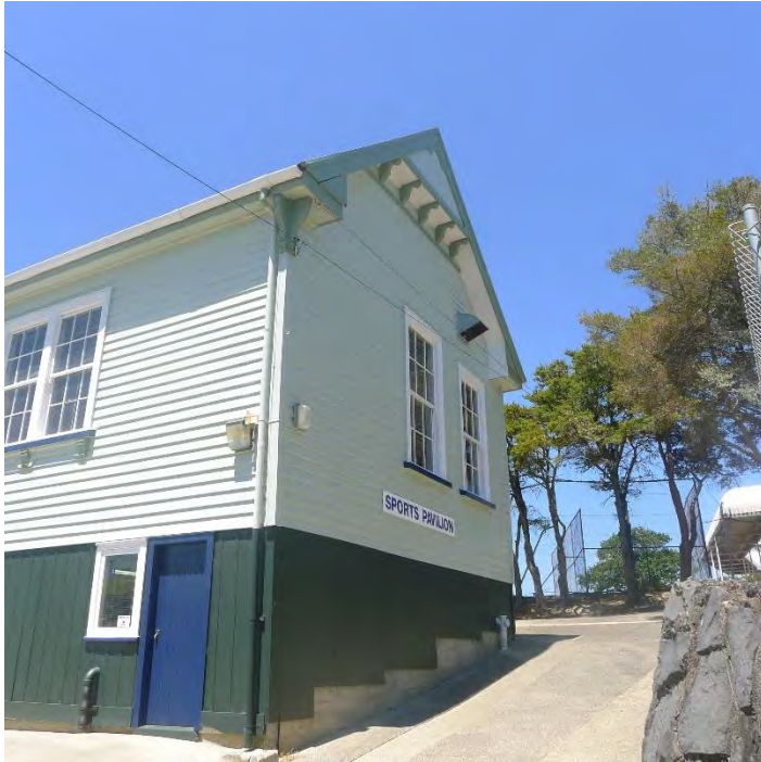
Figure 59: Northcote Public School Infant Department (Former)/Old Gymnasium (Auckland Council; 2013)
