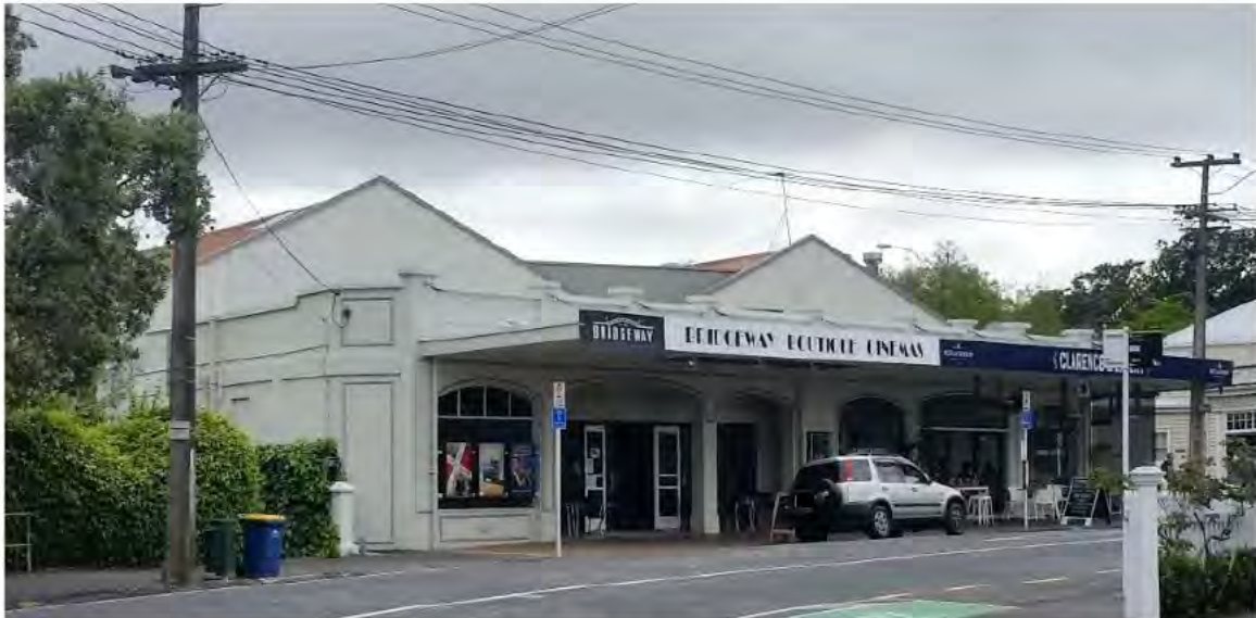
Figure 70: Bridgeway Cinema and Shops (Auckland Council, 28 October 2020).
