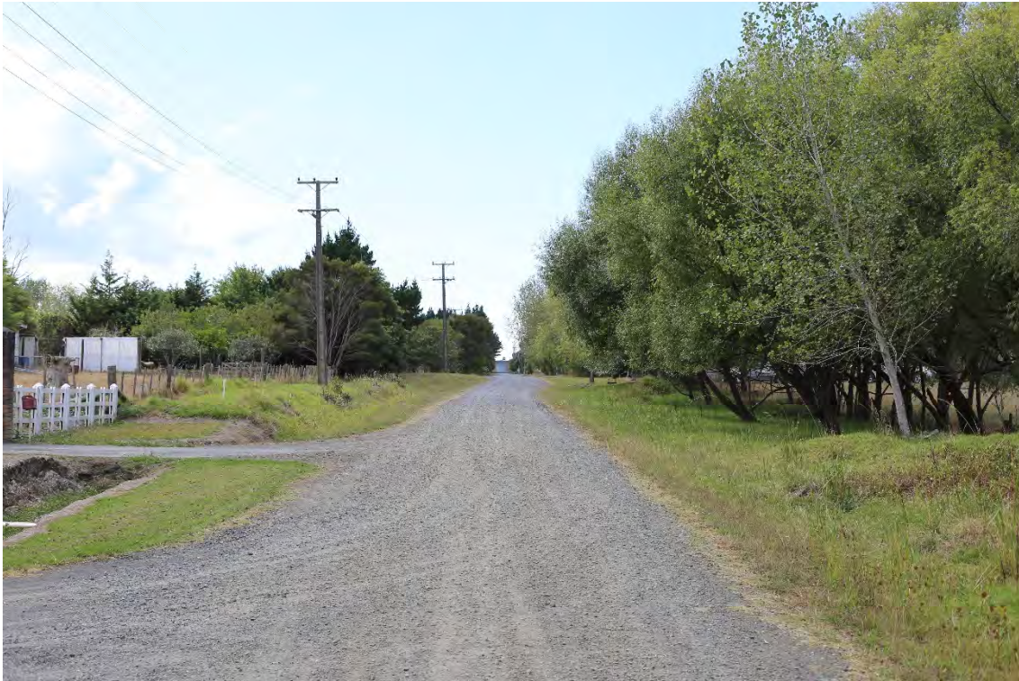
Plate 10. View of Spedding Road condition (looking east)
