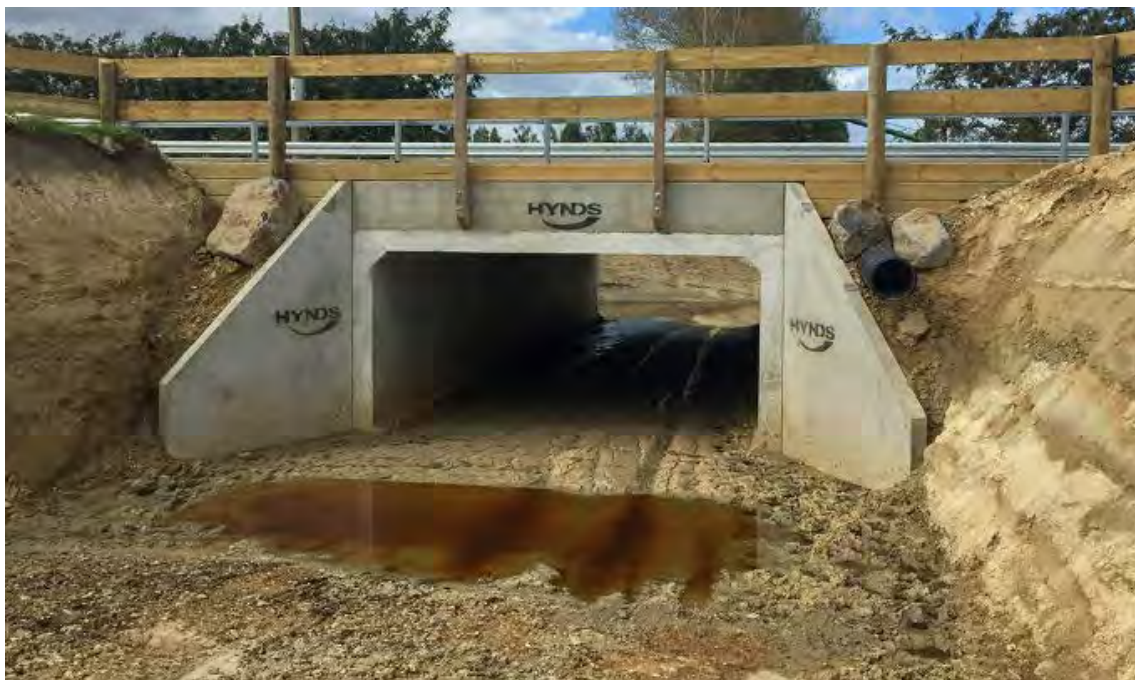
Plate 8. Example culvert, noting that more rip rap and stream flow is anticipated for this Project.
