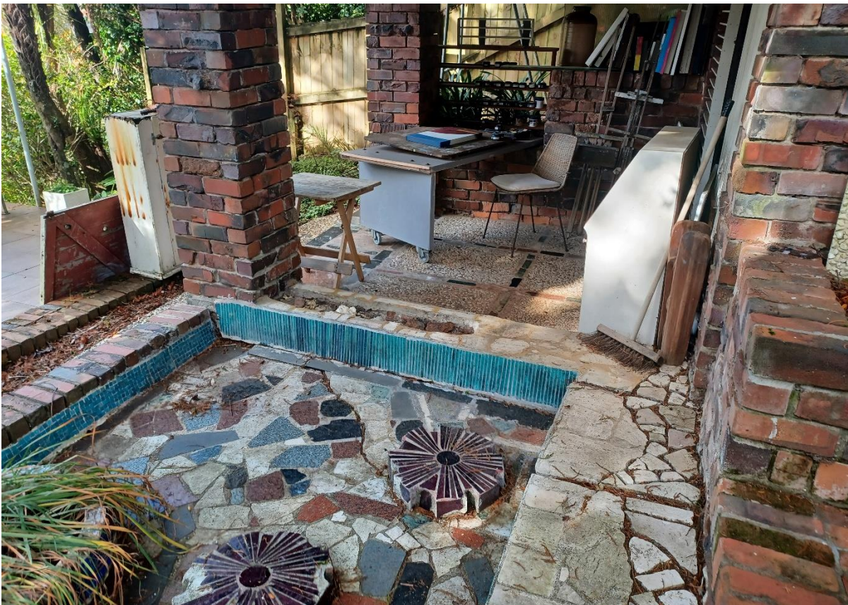
Figure 20: Beneath the studio a small patio is laid in crushed stone, with colour added in embedded tiles. (Auckland Council, May 2022)
