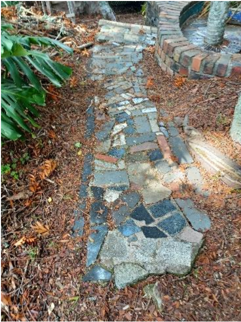
Figure 18 and Figure 19: Glass chips embedded in concrete in the landscaping around the studio and colourful crazing paving of granite and marble on a path next to the studio (Auckland Council, May 2022).
