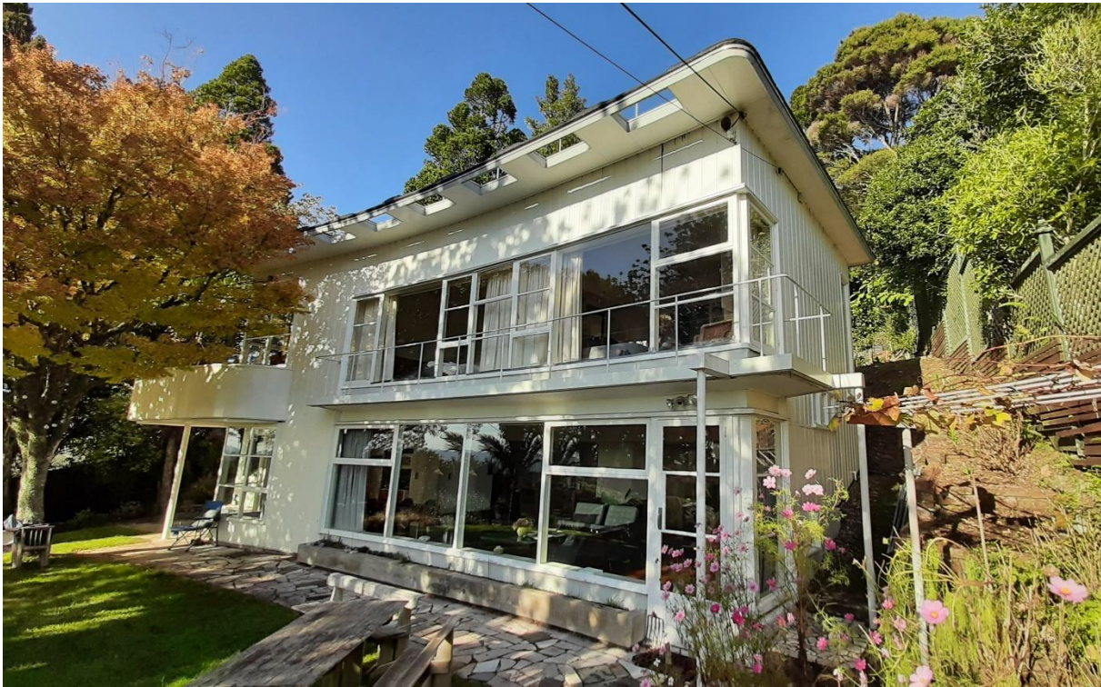
Figure 6: The gently curved front façade (north elevation) of the house featuring large amounts of glazing and access to the front north facing garden. (Paul Jenkin, May 2022)
