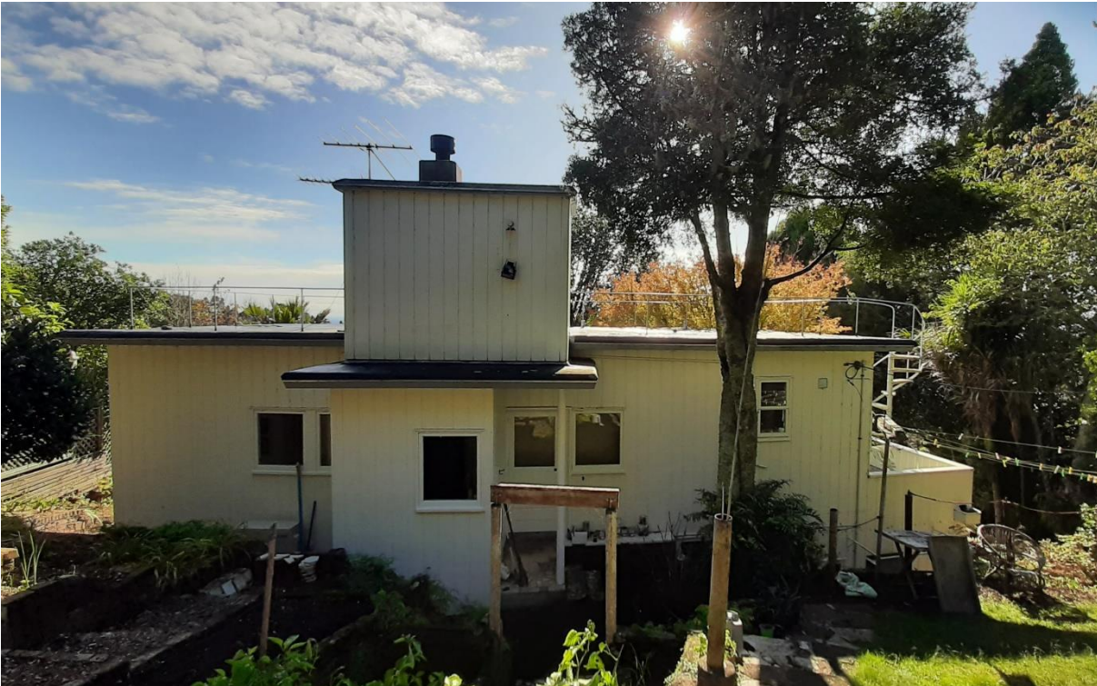
Figure 8: The southern elevation (Paul Jenkin, May 2022).
