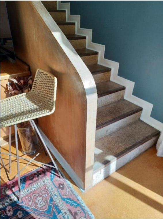
Figure 13 (left): Curved plywood balustrade and cork staircase and Figure 14 (right): Curved ceiling above staircase (Auckland Council, May 2022).
