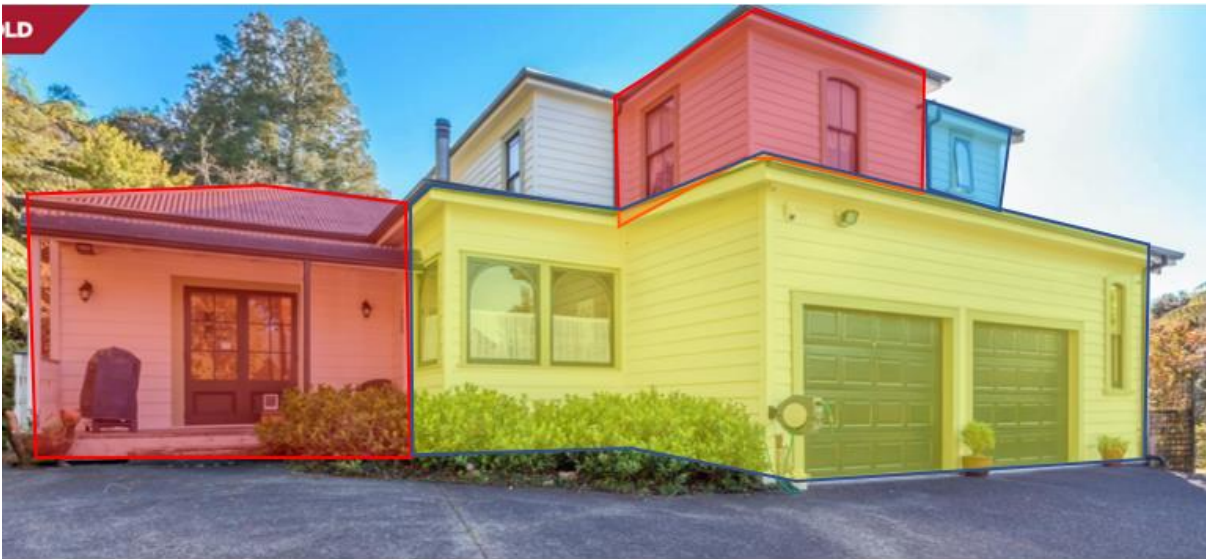
Figure 8: Rear of house showing layers of additions: yellow 1976, red 1993, blue 2011.
