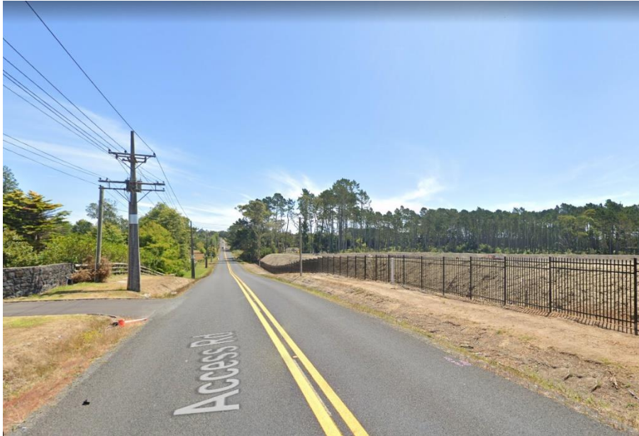
Figure 8-5: Existing Access Road Corridor (Rural Section)
