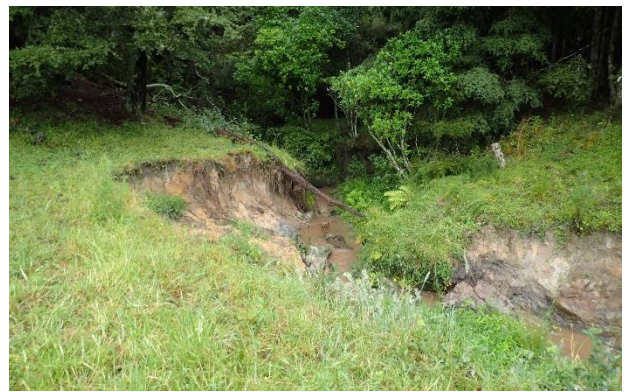
Figure 2. Culvert outlet and adjacent scouring (left) and excessive erosion downstream (right).
