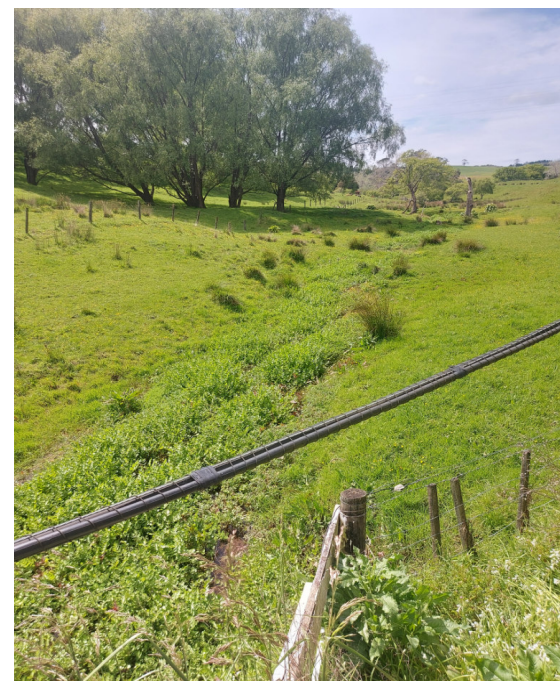
Photo taken during survey looking upstream culvert on SH1.
