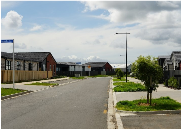
Figure 4-3: New housing development – Maketū Drive, Ramarama (image: Aurecon, Oct. 2023)
