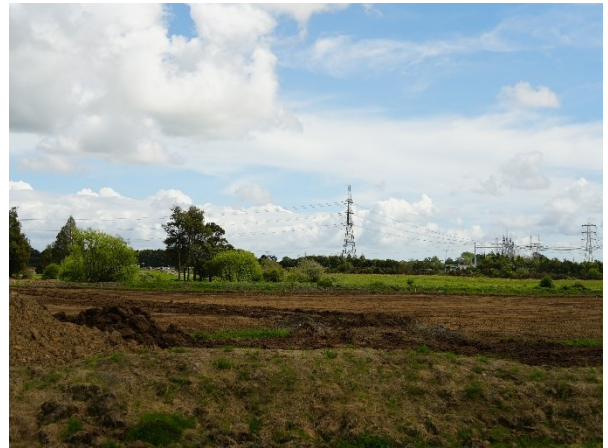
Figure 4-4: Earthworks in greenfield development – Drury South Crossing, Quarry Road (image: Aurecon, Oct. 2023)
