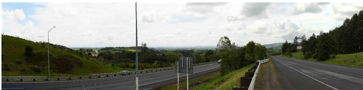
Figure 5-15: Viewpoint 10 existing setting, looking north from GSR parallel to SH1 (image: Aurecon, October 2023)
