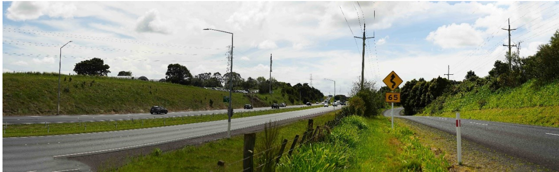
Figure 5-17: Viewpoint 12 existing setting, looking south from Hillside Road parallel with SH1 (image: Aurecon, October 2023)
