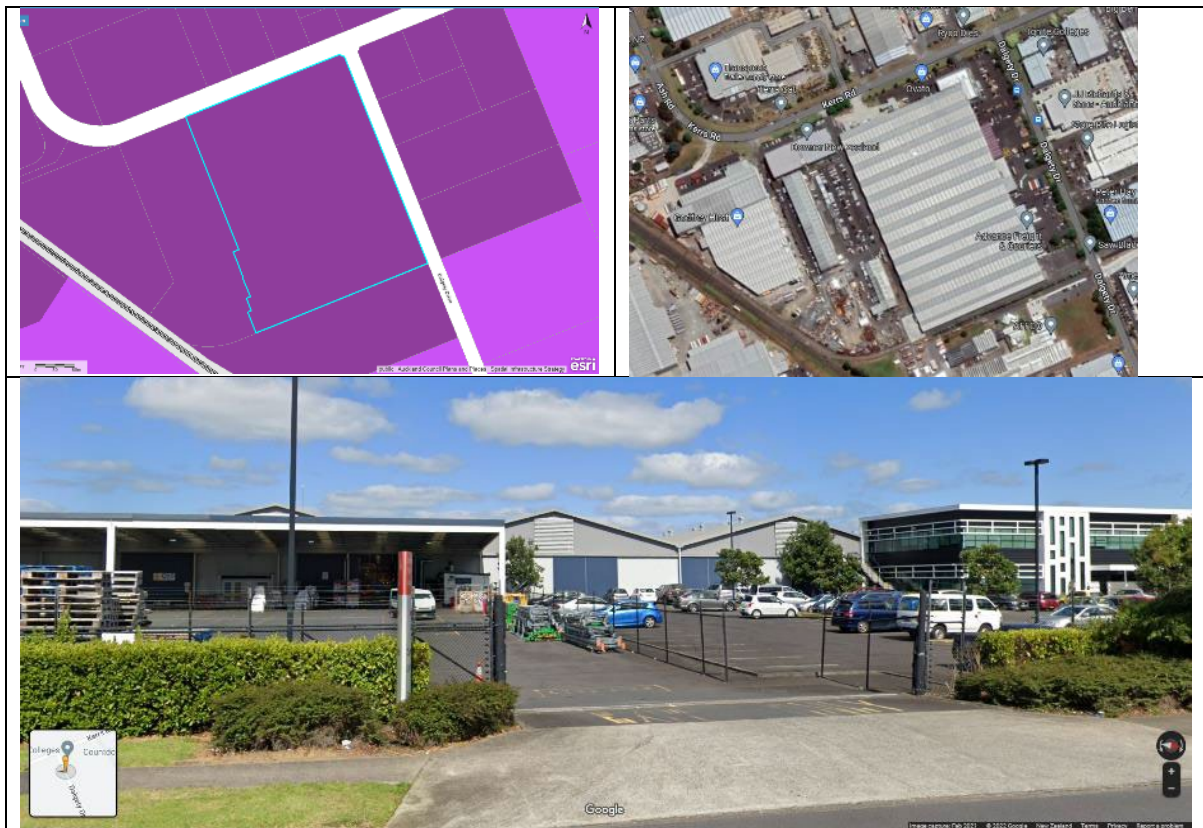
Figure 1: Example of HIZ area, corner of Dalgety Drive and Kerrs Road, Wiri showing large single level building with small corner of building accommodating two levels
