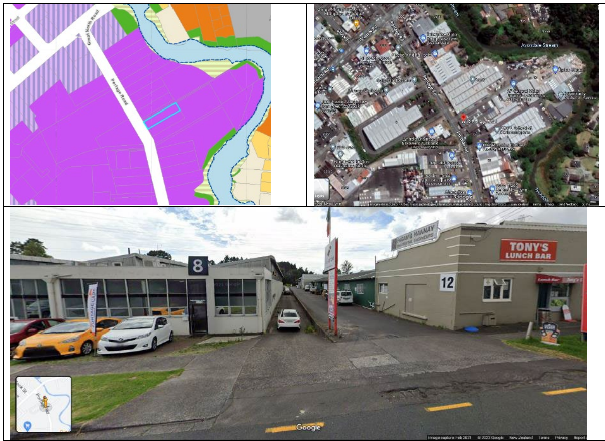
Figure 6: LIZ area in Portage Road, New Lynn showing motor vehicle sales, older industrial units and small food and beverage/lunch bar
