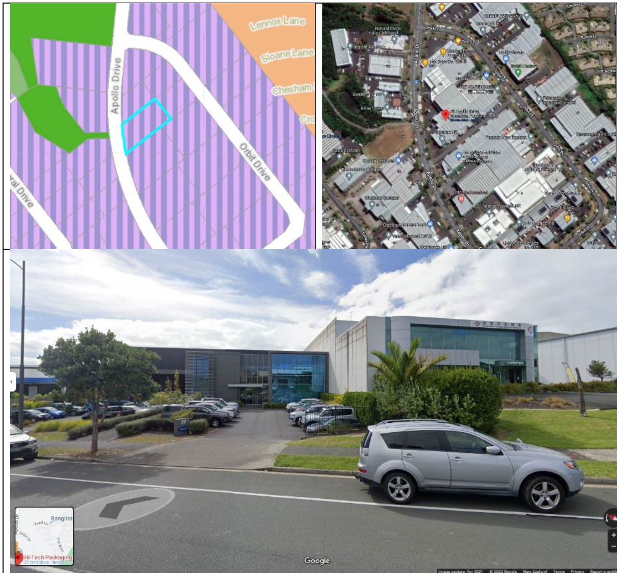
Figure 8: Example of GBZ at 79 Apollo Road, Rosedale.
