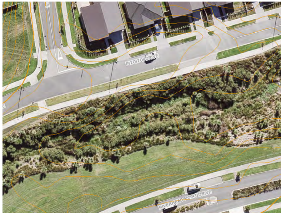
drainage corridor/swale along Riverhead Point Drive
