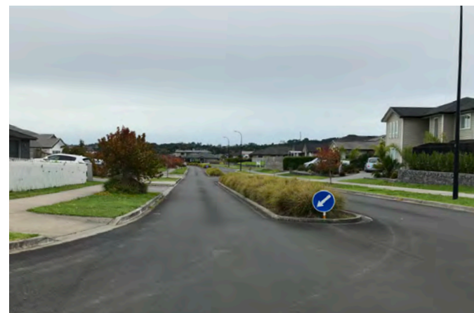
Central swales in Riverhead Point Drive
