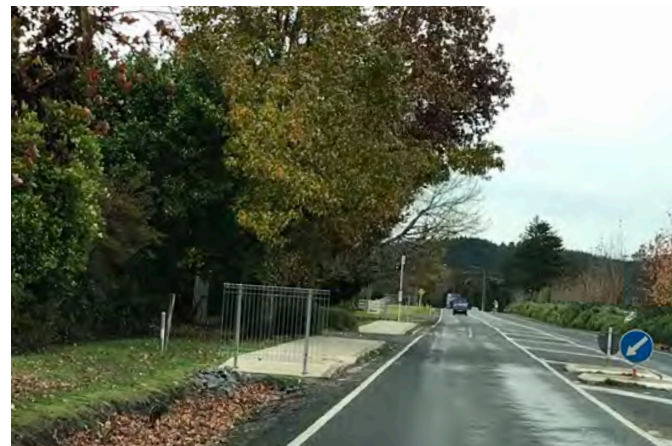
Coatesville-Riverhead Highway (alongside Grove Way)
