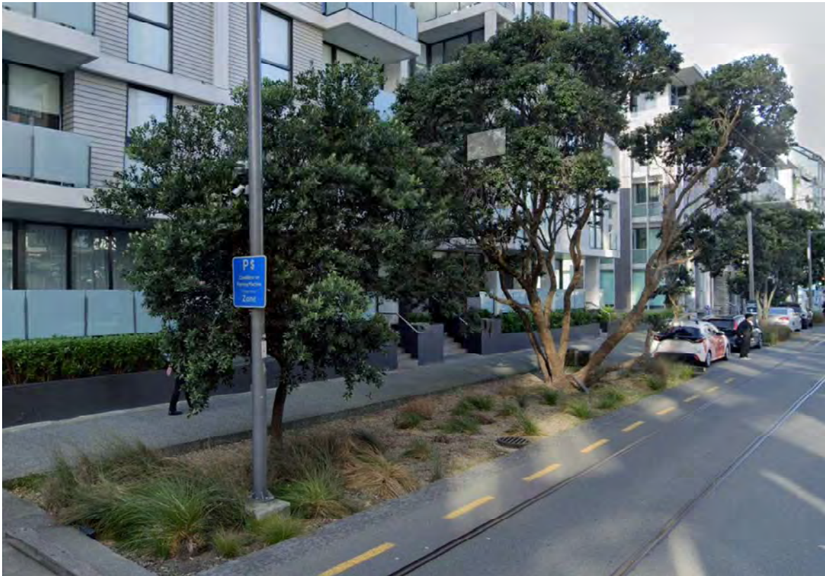
Figure 7. Example of a Raingarden (Halsey Street Auckland CBD)
