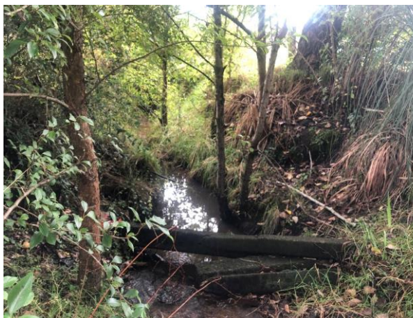
Photo 3: Concrete beams spanning the channel of watercourse 2.
