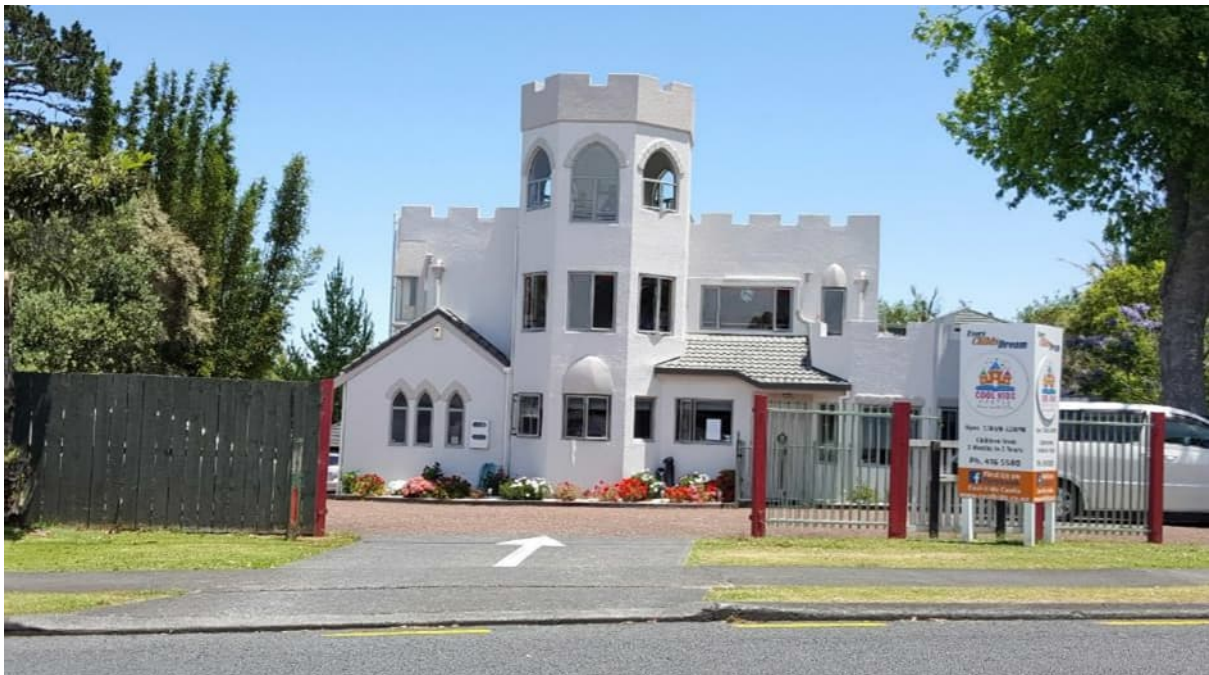
Figure 21: 5 Luckens Road (childcare centre) (source: Macready 2019)
