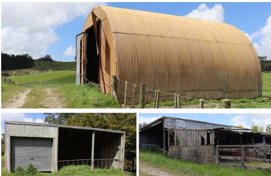
Figure 30. Top: large rounded corrugated iron shed located on central north side of property, facing east. Bottom left: shed located on central south-east side of property adjacent to central stream, facing south. Bottom right: shed located on central west side of property, facing southwest
