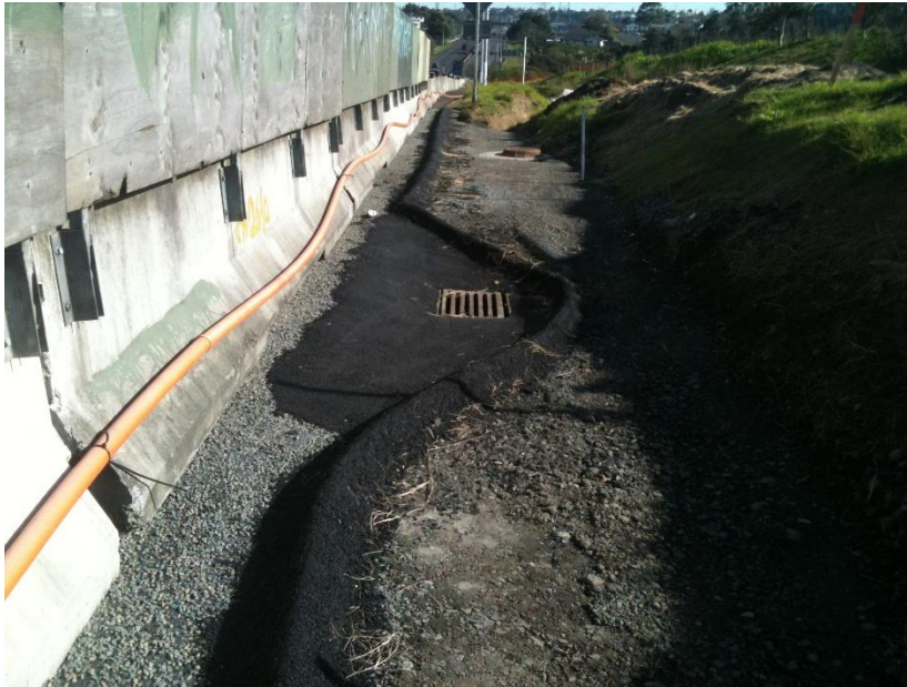
Photo 2: Hotmix Bund used to divert existing road runoff and separate works area, used on the North-Western Motorway.
