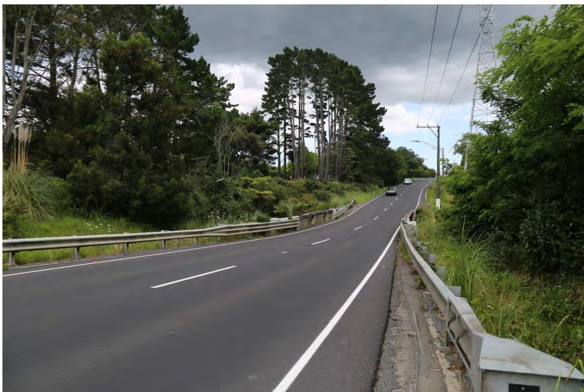
Figure 9-4: View west across the Totara Creek Bridge along Brigham Creek Road.
