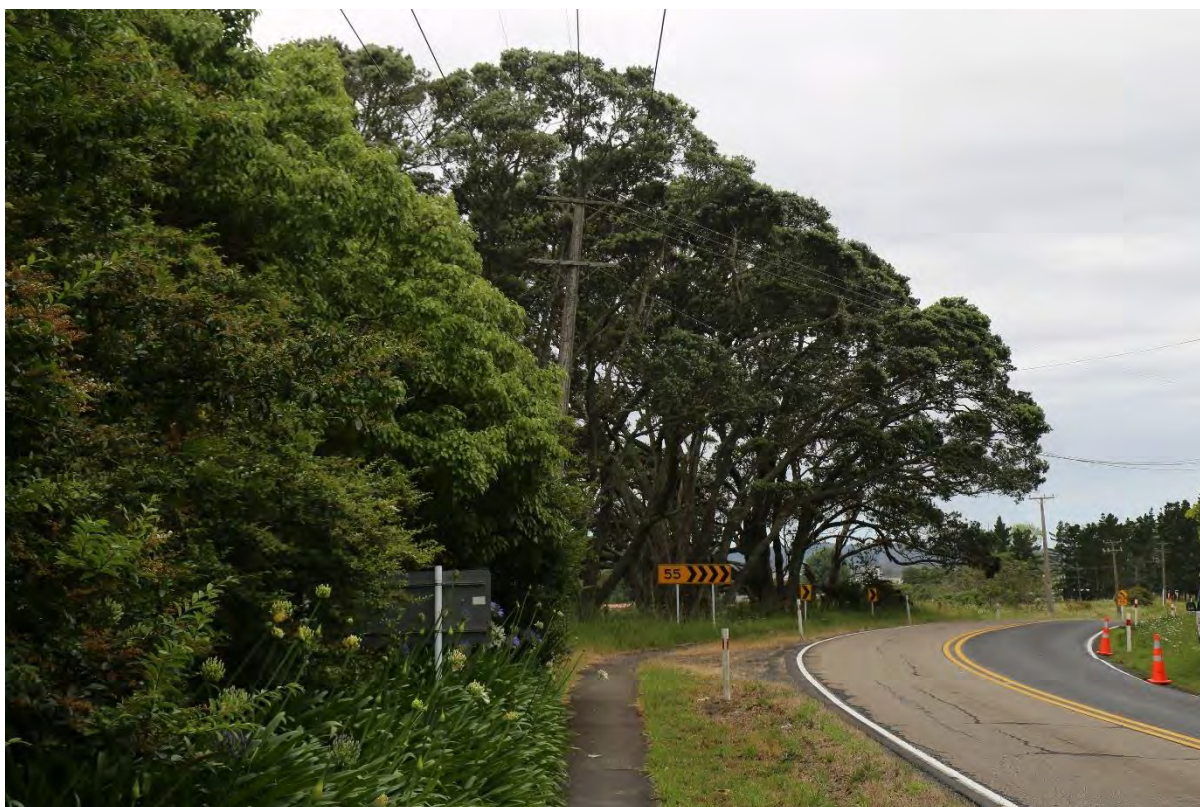
Figure 7-1. View north along the road corridor from outside of 92 Trig Road.
