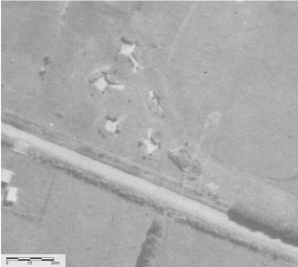
Figure 32: The gun emplacement in 1959 with some of the buildings already demolished but all gun pits still clearly visible.
