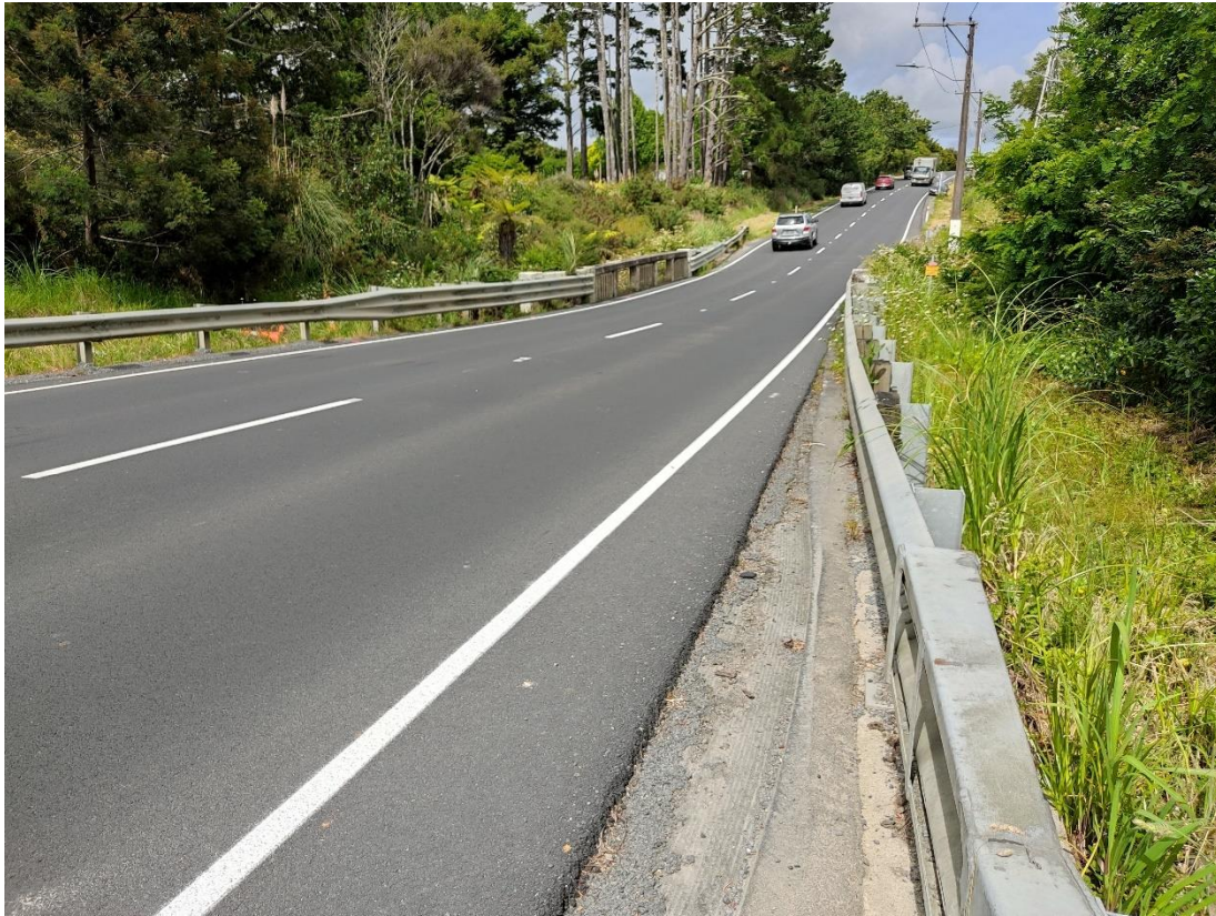
Figure 20: Narrow bridge over the Totara Creek.
