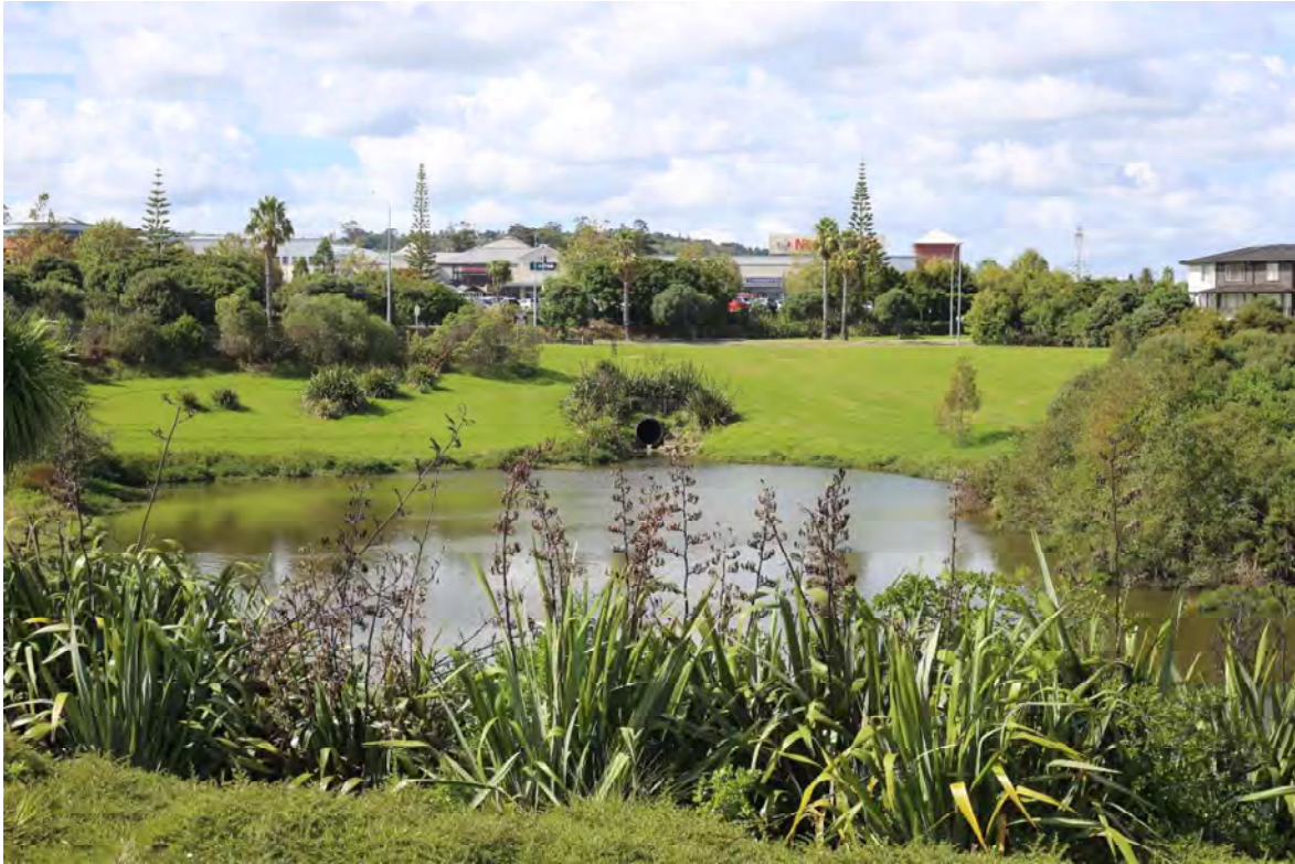
Figure 5-5. Whaka Maumahara stormwater pond and culvert beneath Te Irirangi Drive
