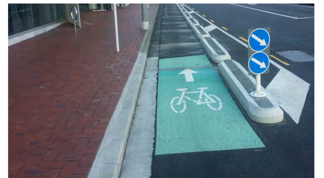
Upgrade Coatesville-Riverhead Highway and Riverhead Road to provide new and safe facilities for pedestrians and cyclists, providing local residents with genuine travel choices
