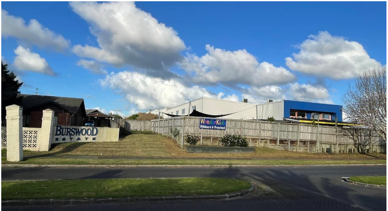
Figure 21. North and west-facing walls of Wonderkids Childcare and Preschool (location D); imagery from Google Maps Street View looking east from 200 Burswood Drive, photo taken 16 May 2023.
