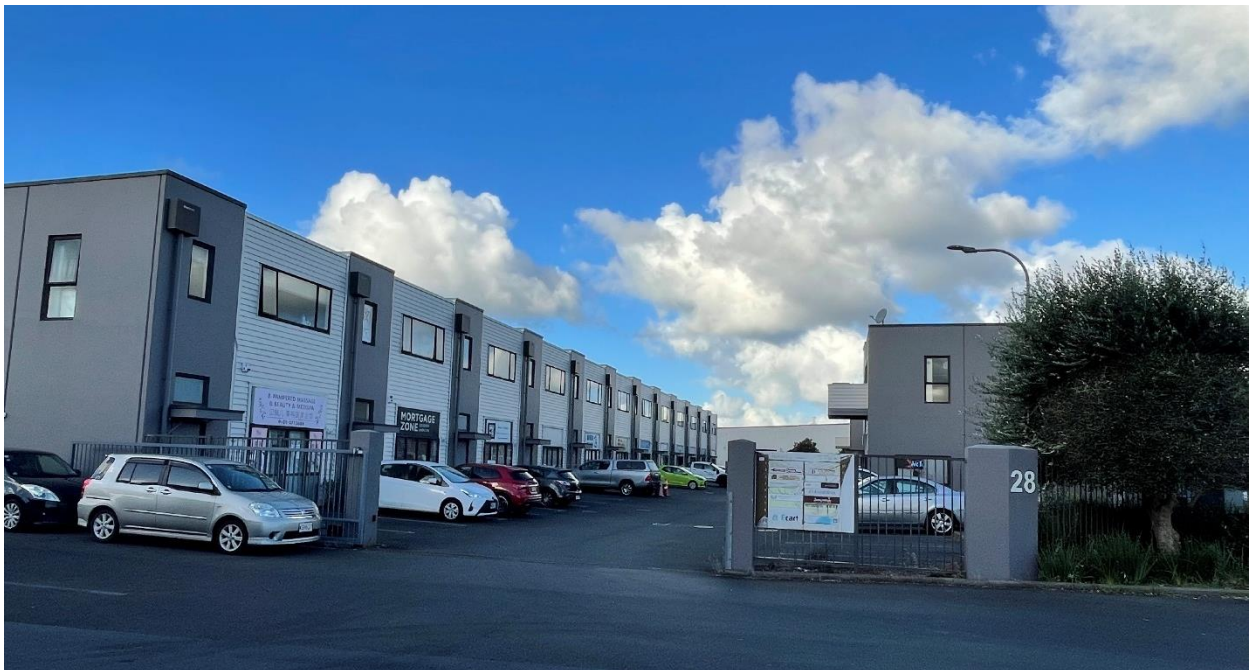
Figure 18. Location B – 28 Torrens Business Park (commercial/residential units). Upper image – north-facing profile. Lower image – south-facing profile; photos taken 16 May 2023.
