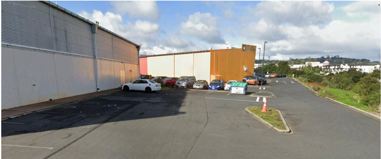
Figure 29. Location K –west-facing walls of tyre workshop (centre) and other retail buildings in The Hub (left). Image looking south, Guys Reserve shown at right of image; imagery from Google Maps Street View, image taken July 2022.
