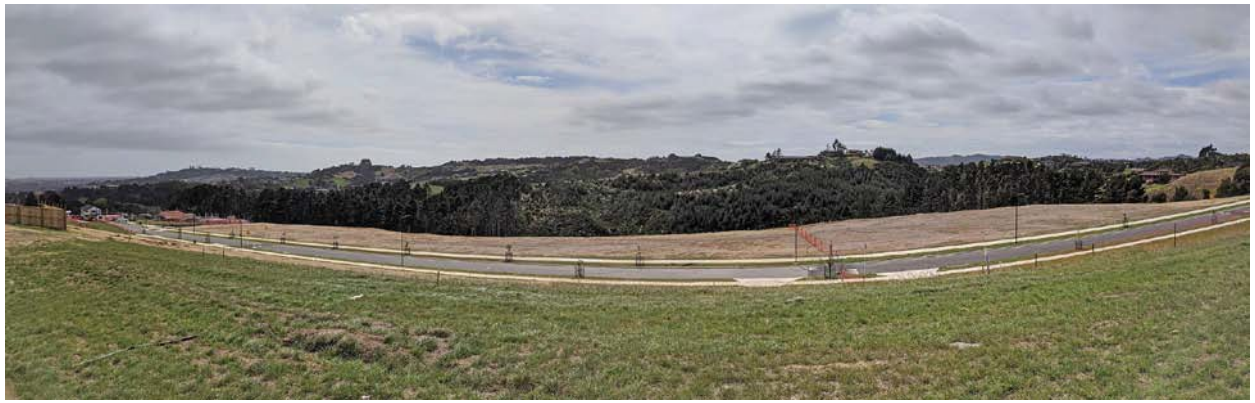
Photograph 7 Redoubt Road Ridge seen from Michael Bosher Way. The RPO lies in the bottom of the valley beyond the edge of the earthworks.
