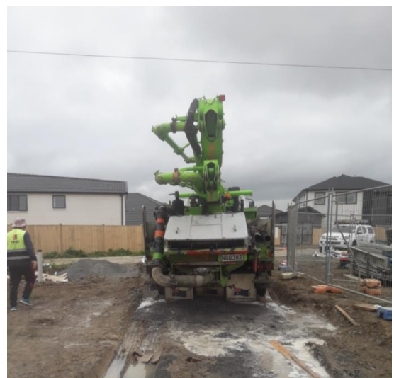
Photo 1: Concrete pump truck parked beneath National Grid transmission lines
