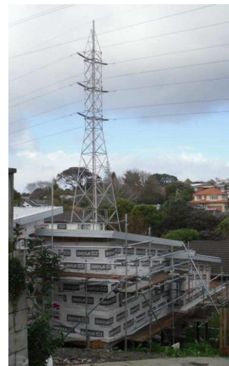
Photo 2: New dwelling blocking access to Tower 48 HEN-ROS line
