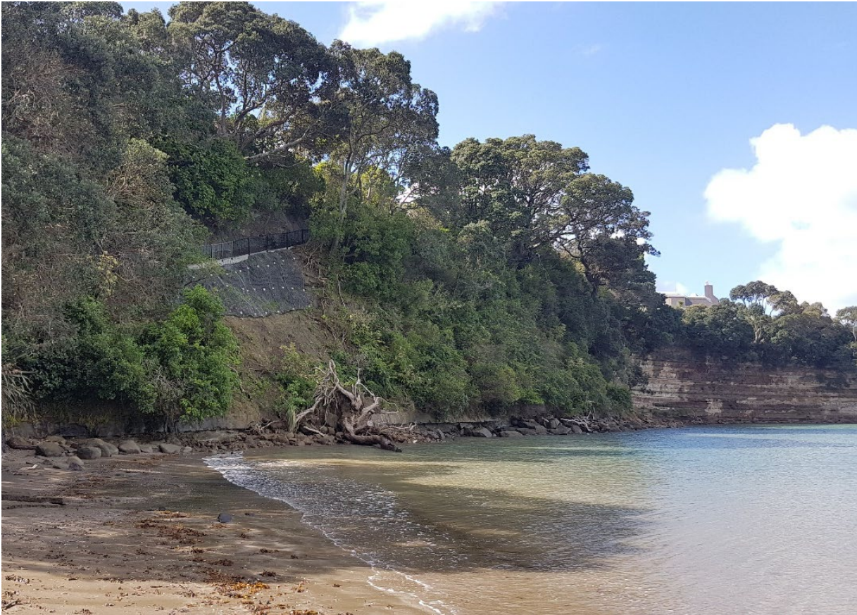
Figure 2: A typical Auckland East Coast cliff showing a recent repair to reinstate a footpath damaged by cliff instability As the toe of these cliffs is eroded, instability higher up the cliffs will increase.
