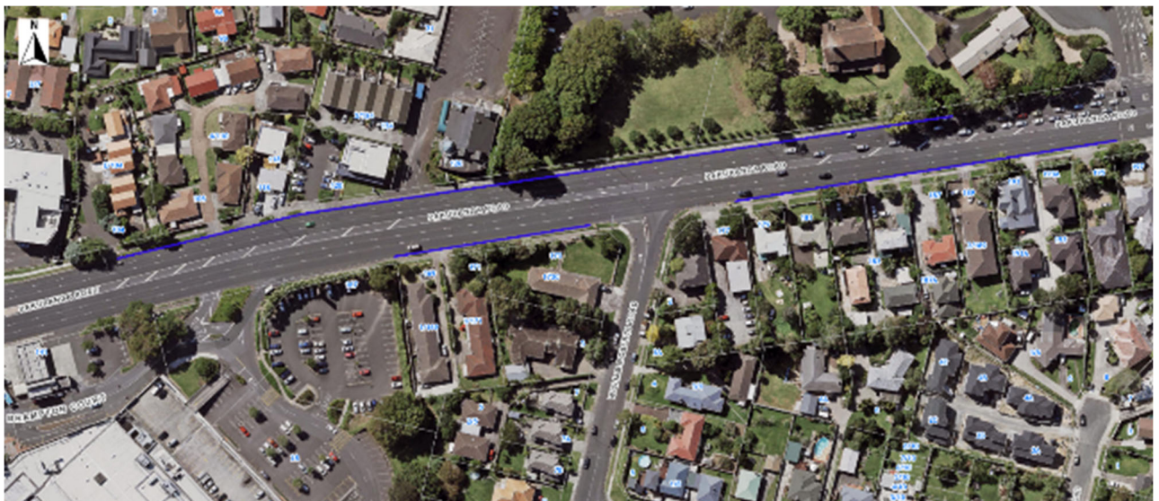
Figure 83: Pakuranga Rd clearways and on-street parking (blue outline)
