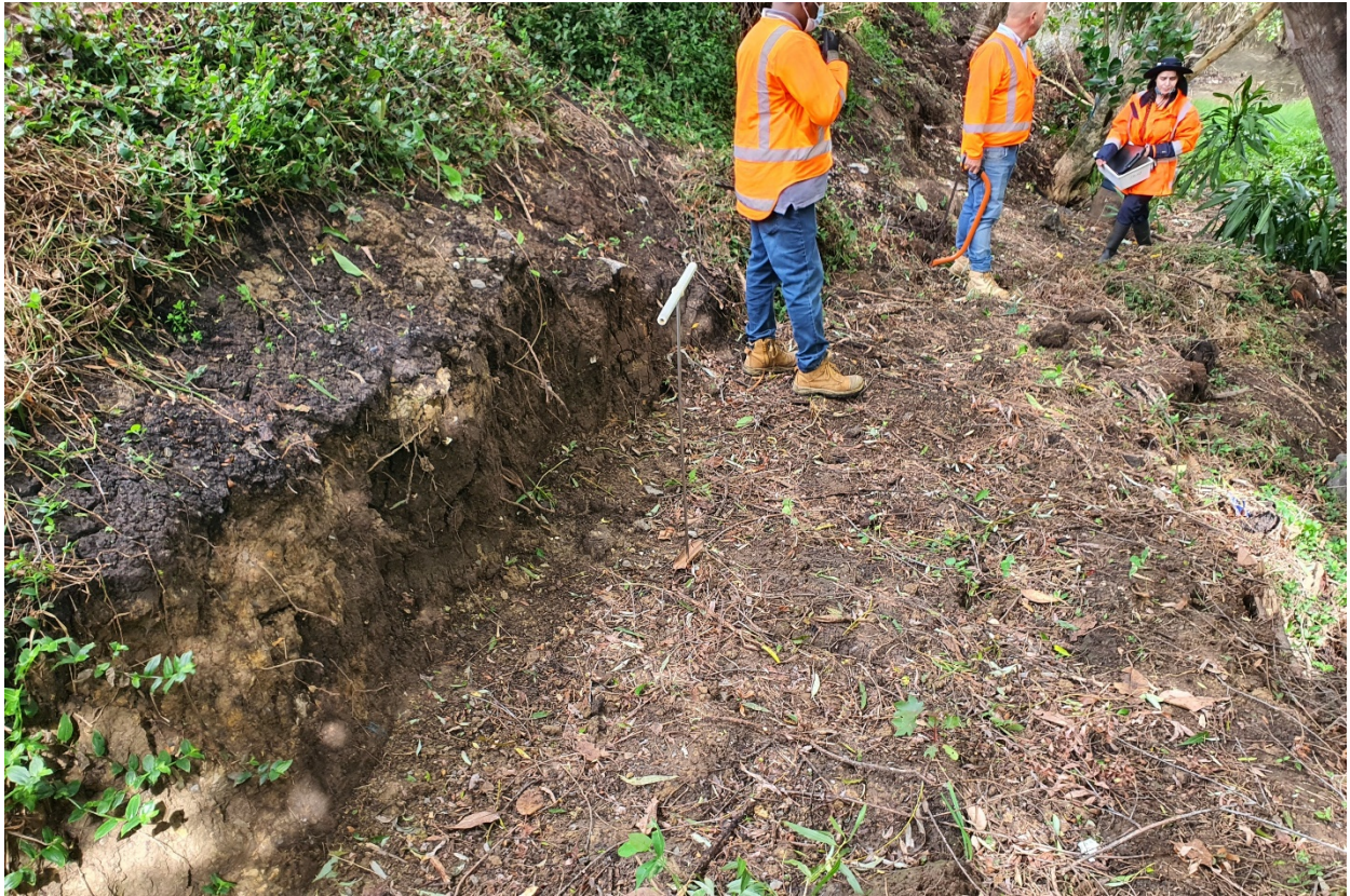
Figure 12. cut made for digger access showing up to 1 m of fill.
