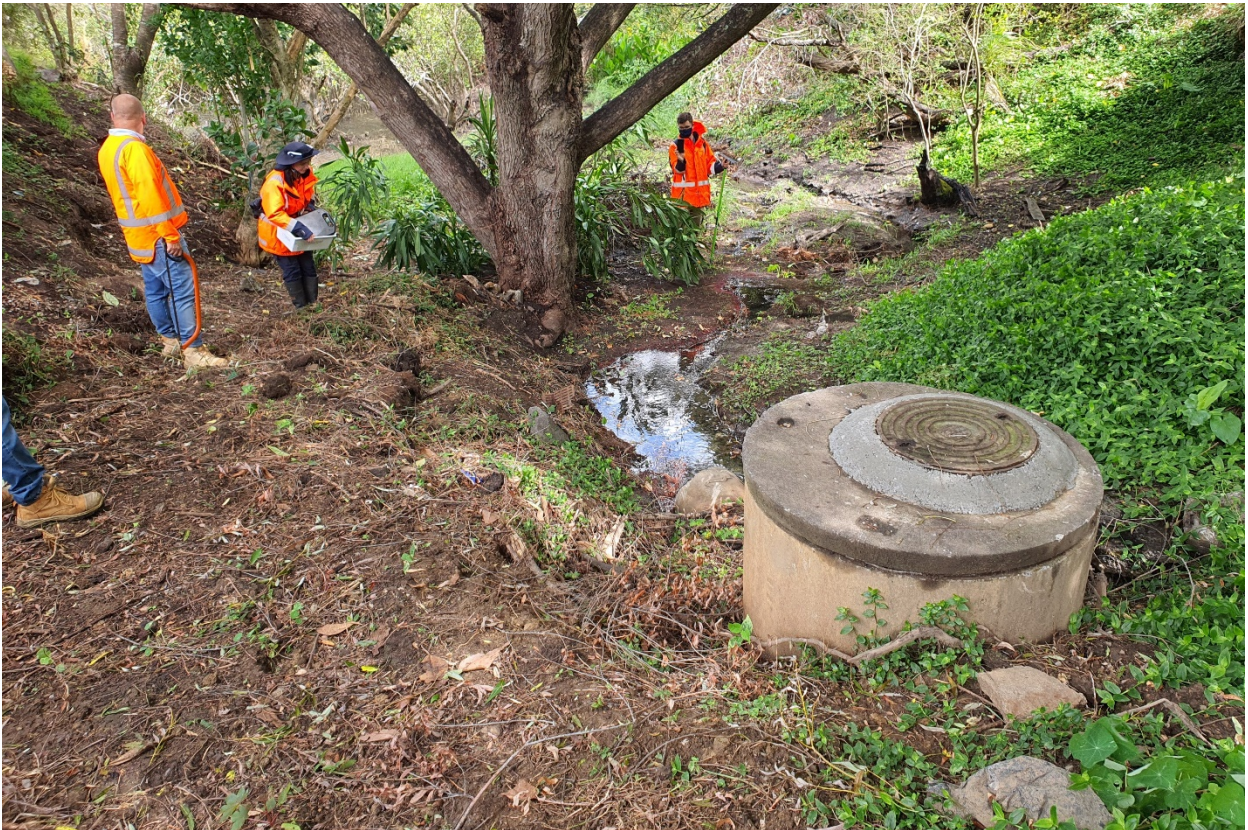
Figure 11. Recently cleared area around MCC_108738 for stormwater upgrades.
