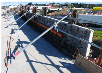
Bridge edge barrier installation
