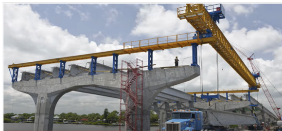
Beam gantry launcher
