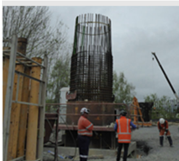
Piling & pile cap construction
