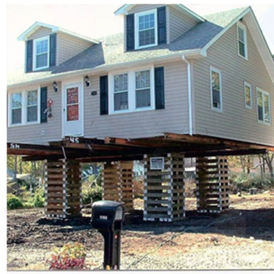
House on temporary bearers
