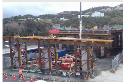
Temporary works for superstructure
