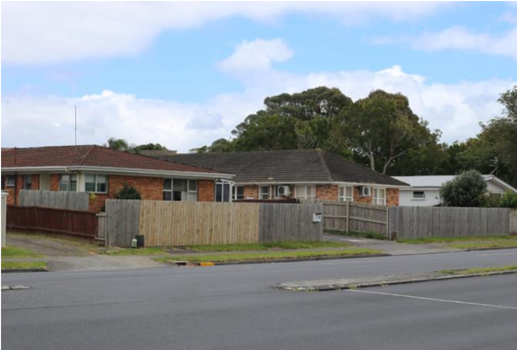
Figure 6-5 Typical Housing on Ti Rakau Drive
