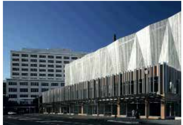
Parking building with an active retail ground floor – Auckland City Hospital
