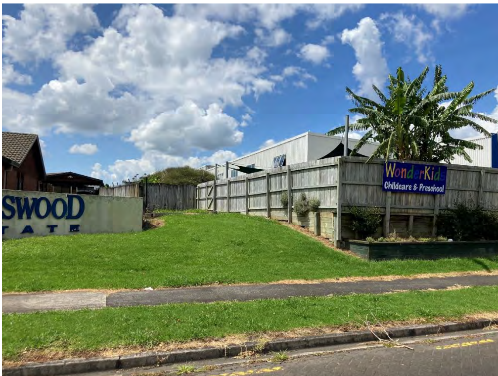
Image showing the rear of WonderKids Childcare and Preschool and the existing berm area. View from Burswood Drive
