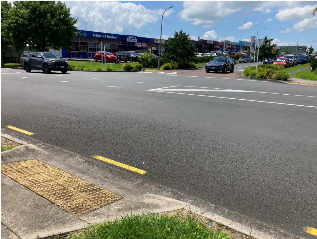
Image showing intersection of Burswood Drive and Torrens Road and current informal pedestrian crossing
