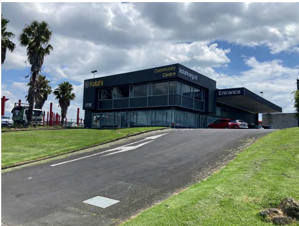
Image showing the Kotahi community centre entrance at 272 Ti Rākau Drive
