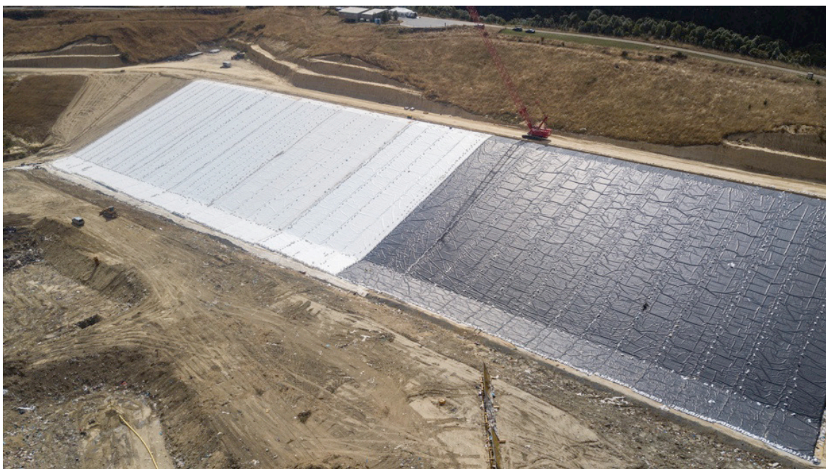
Above: Transfer Station Below: Cell Lining
