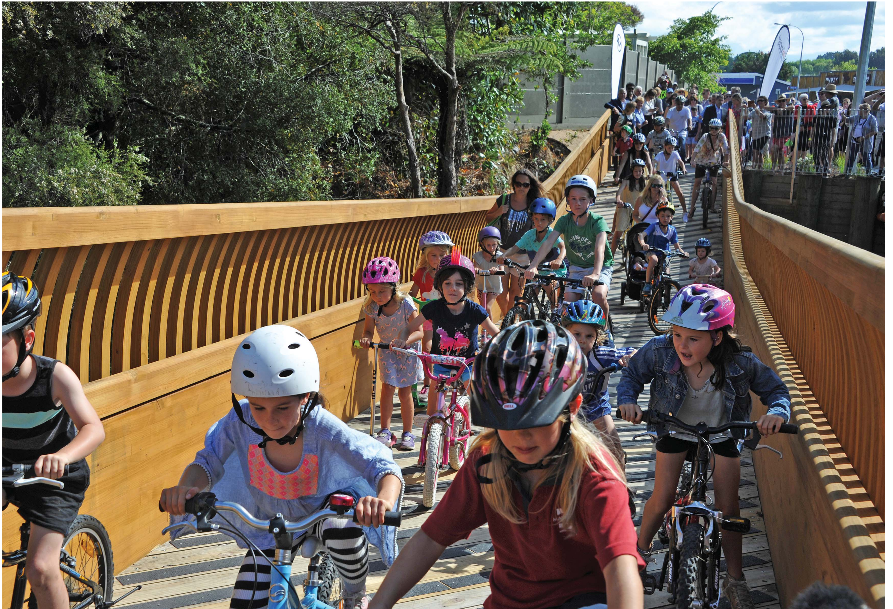
Matakana Village cycleway bridge opening, 2016
