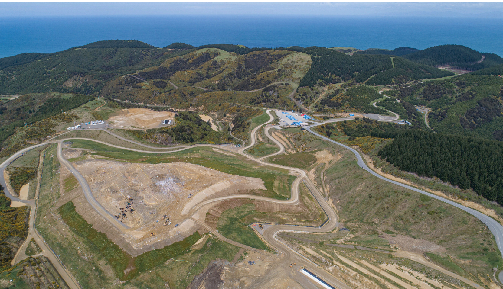
Big picture of operations. Gas on the left and Transfer on the right.
