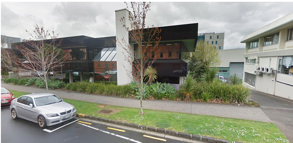
Figure 3: The office building at 47 George Street. At the right of the picture is the ACG Primary School, behind which is an existing building on the Precinct site and, in the background, the new Mercury Energy Building at 33 Broadway.
