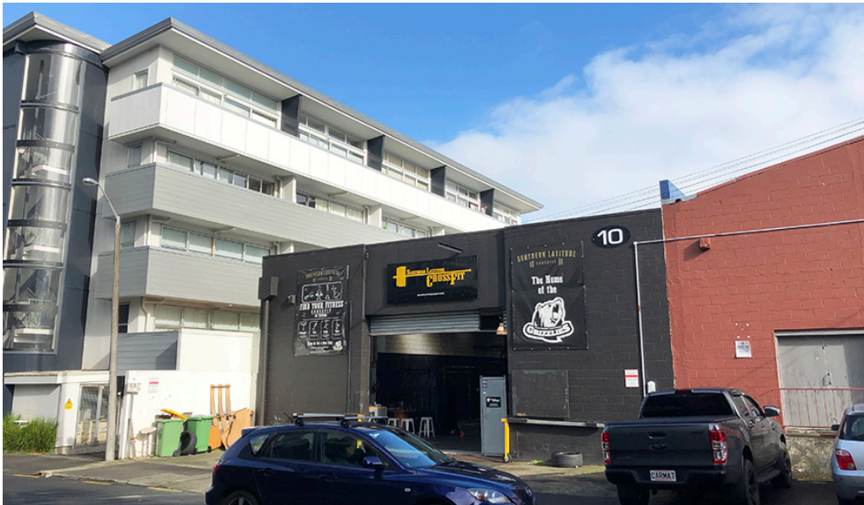
Figure 9: Looking towards the apartment building at 8 Clayton Street, with the existing gym within the Precinct site (10 Clayton Street) in the foreground.
