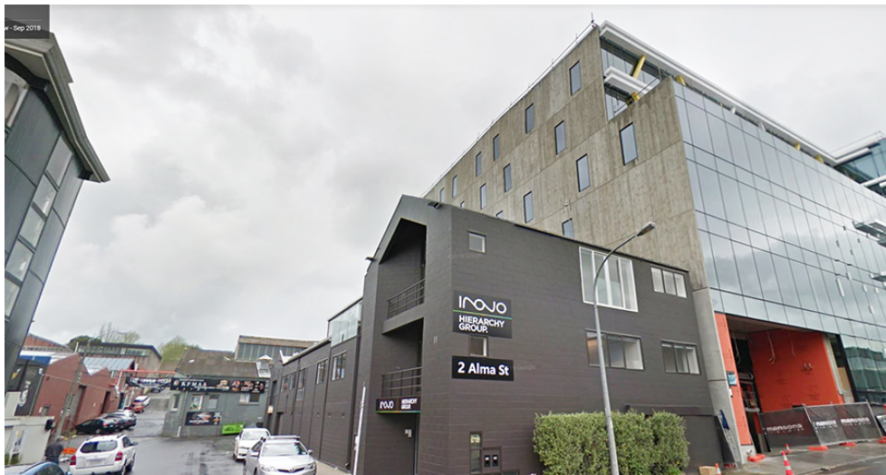
Figure 10: Looking north along Clayton Street, through to the existing driveway into the Precinct site. 2 Alma Street is at the centre of the photograph, with the new Mercury Energy Office building behind it.
