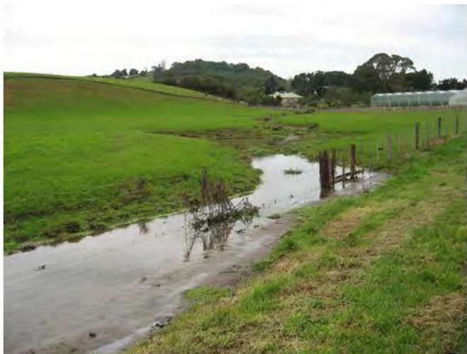
LOCATION F (FIG2)-The southeastern stream ponding behind a road culvert, 50 metres downstream of the proposed Willow Road Re-alignment
