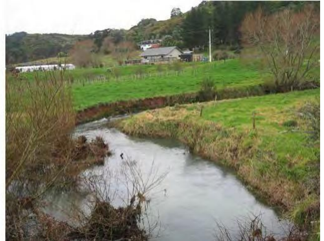
The Maketu channel with erosion scour at the outside bank
