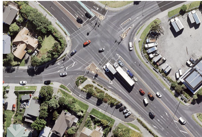
Intersection of Schnapper Rock Road, Albany Highway and Bush Road
