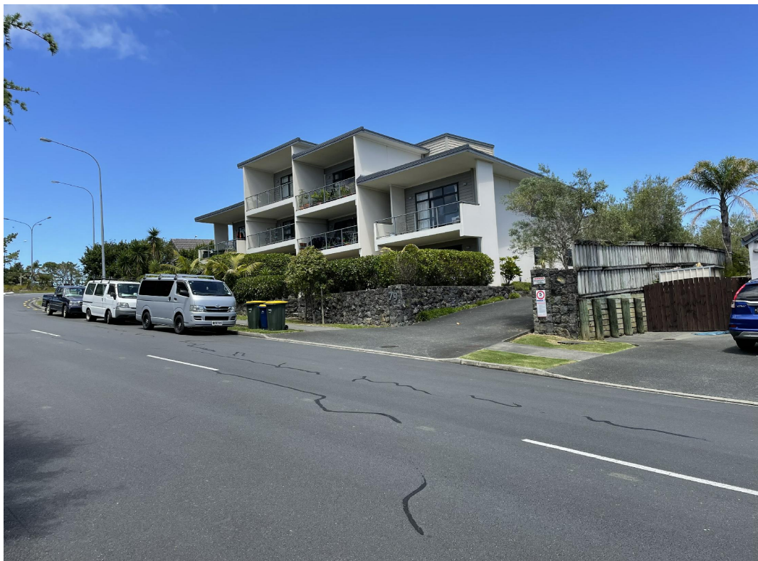
Three storey apartment
