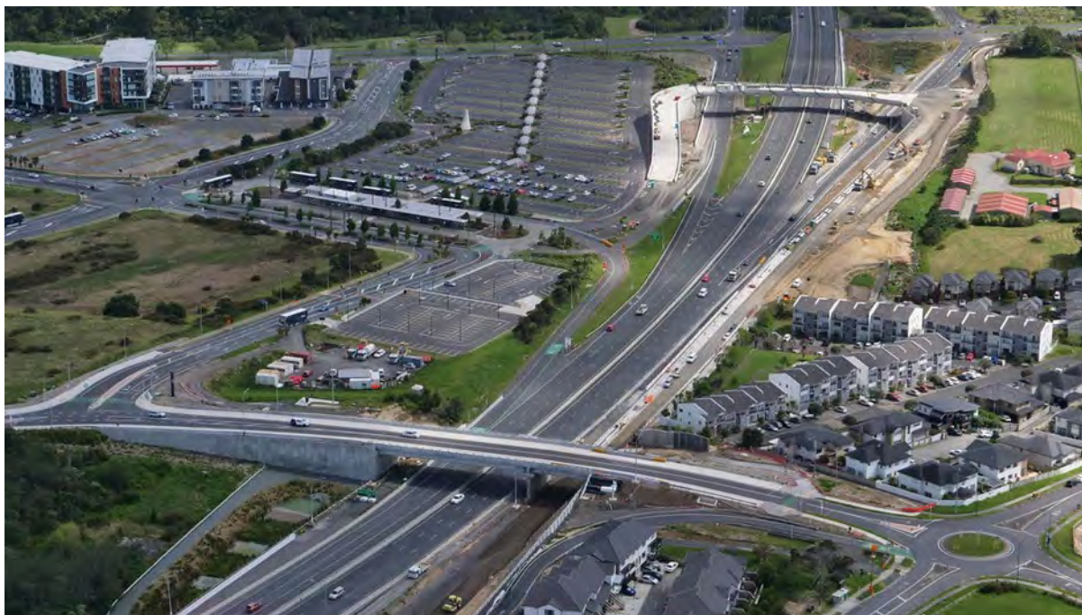
Image 4 - October 2021 Waka Kotahi photograph 4 of progress at the Albany Busway Station and associated walkways and cycleway progress linking to eastern side Oteha Valley Road
