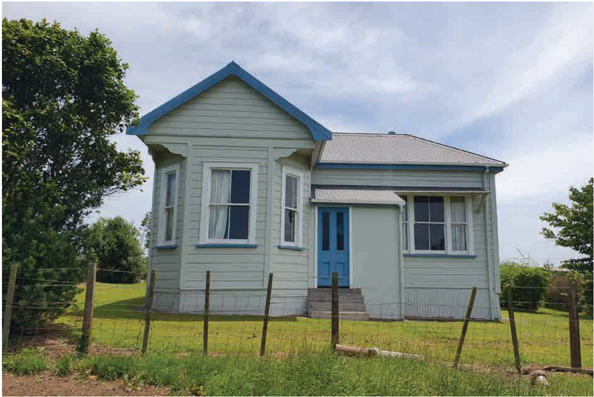
Figure 6. View west of front of Villa.
