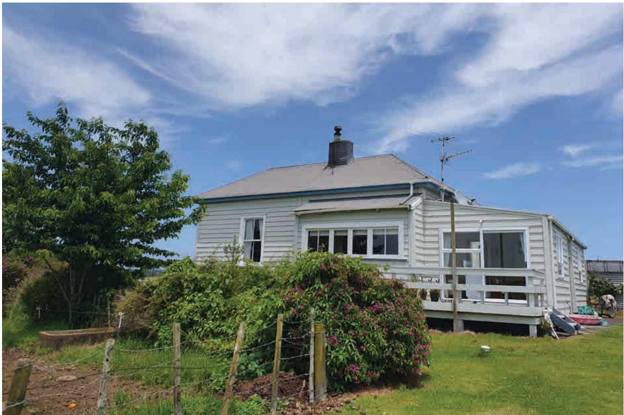
Figure 7. View south east of house showing additions on north western side.
