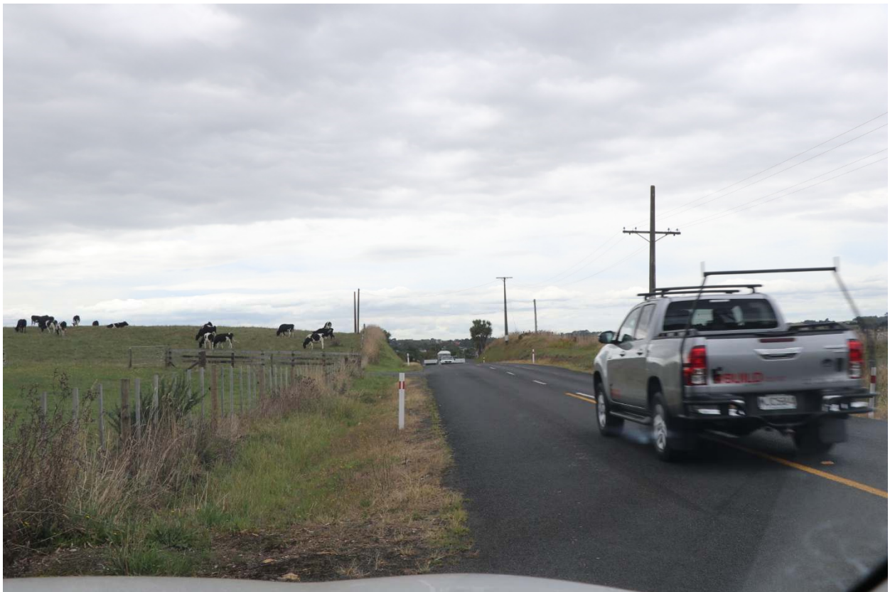
Figure 11: Southern Intersection Visibility to the North (120m)
