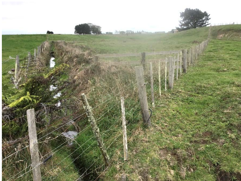
Figure 8: Constructed drain on boundary of 130 Constable Rd (92 Constable Rd to left of image).
