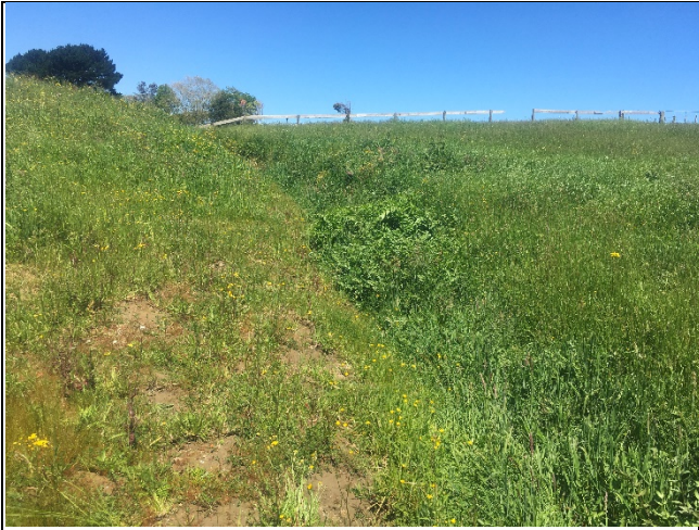
Drainage feature – view south east, or upstream.
