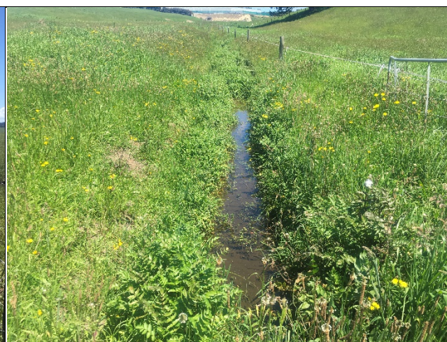
Drainage Channel – view south-west.
