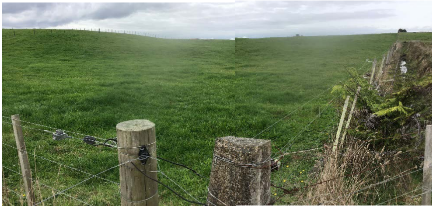
Figure 5: Area mapped as overland flowpath in western quarter of 92 Constable Road.
