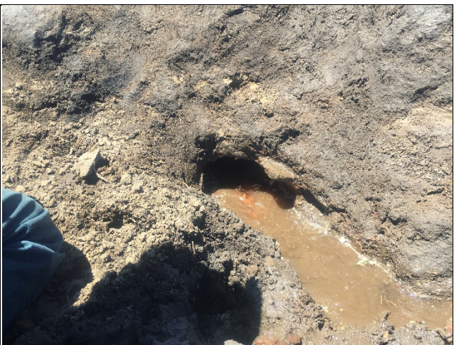
Drainage feature outlet showing the visible pipe.
