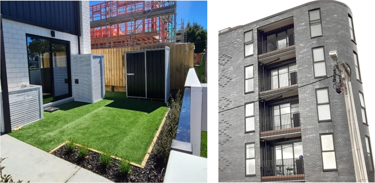
Figure 21: The useable space of the ground floor outdoor living area is reduced by the presence of a heat pump, shed and water tank. In this site, the items are screened. The useable space on the balcony in the apartment building is reduced by the external heat pump unit.
