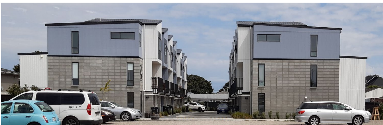
Figure 18. This three storey terrace development shows the outdoor living spaces (in the form of a balcony on the first level) and principal outdoor living space taking advantage of the driveway space to meet the AUP standards. The AUP requirement for sunlight to outdoor living spaces plus the requirement for a 6m outlook space from the living area has caused the 6+m wide driveway to be located in the central core of the development. The outlook spaces and outdoor living spaces (balcony) of each terrace block face each other across the driveway which can affect privacy.
