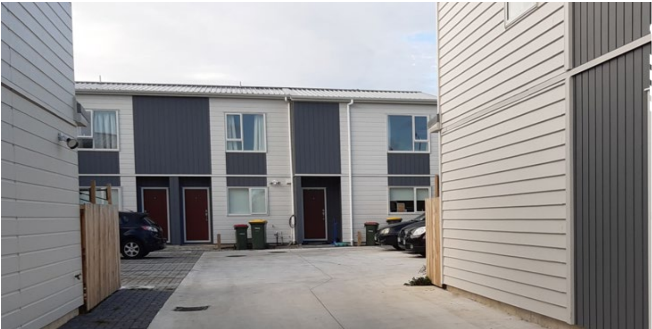
Figure 31. Development with front doors opening directly onto a communal parking area and vehicle manoeuvring space. The designated footpath area (dark grey paving adjacent to the dwelling on left), directs pedestrians into the reversing space of cars enroute to the front doors of dwellings.
