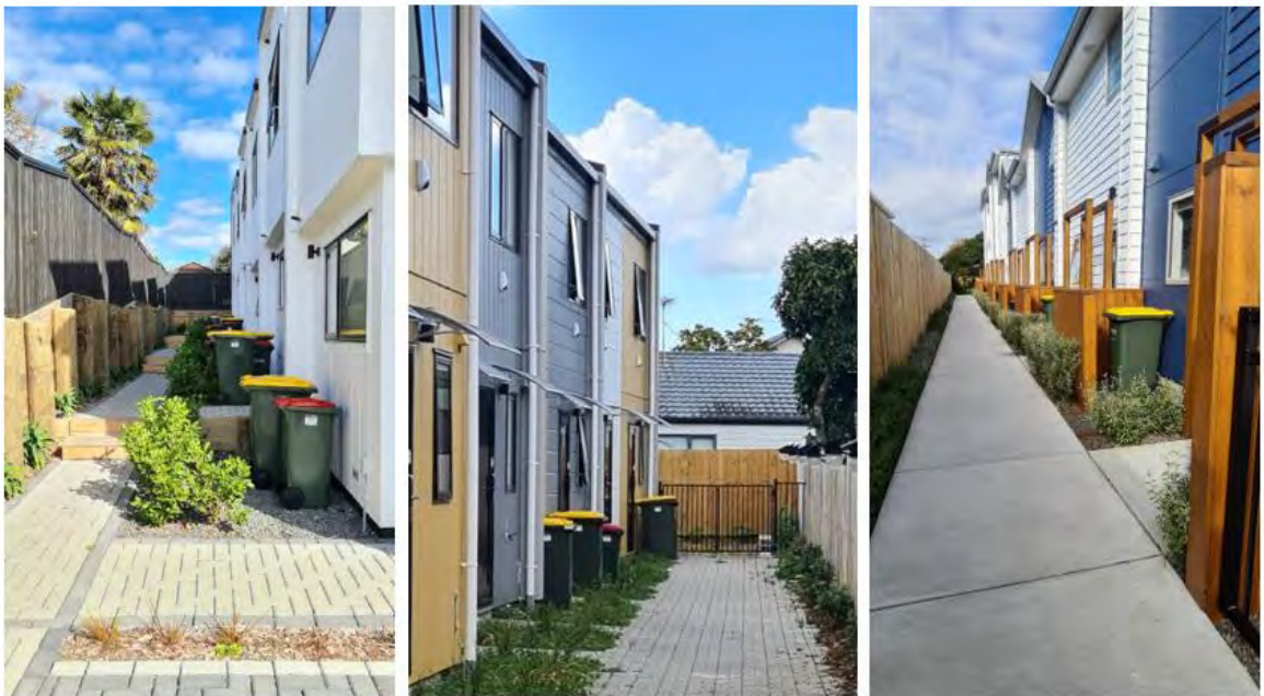
Photos 19, 20 & 21: Individual waste bins stored adjacent to pedestrian access routes to dwellings
