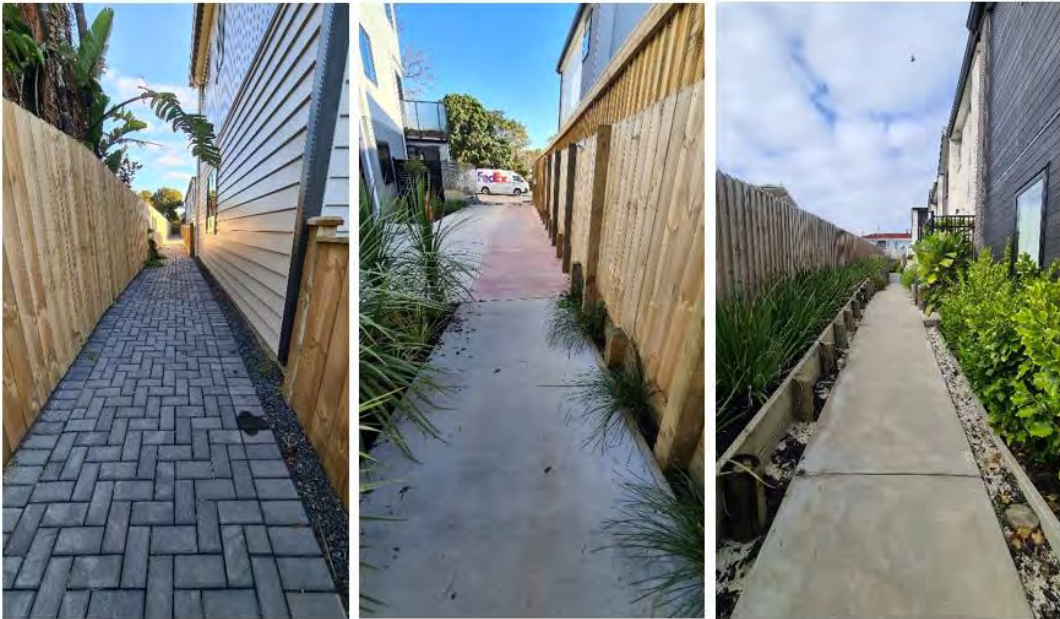
Photos 14, 15 & 16: Examples of landscape buffers between footpath and dwellings
