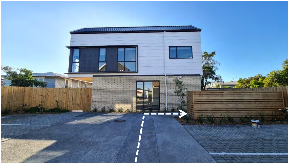
Photo 1: Seven unit development in Henderson 11 - Pedestrian access route to dwellings extends behind carparks and dog-legs around communal bin enclosure (white dashed line)
