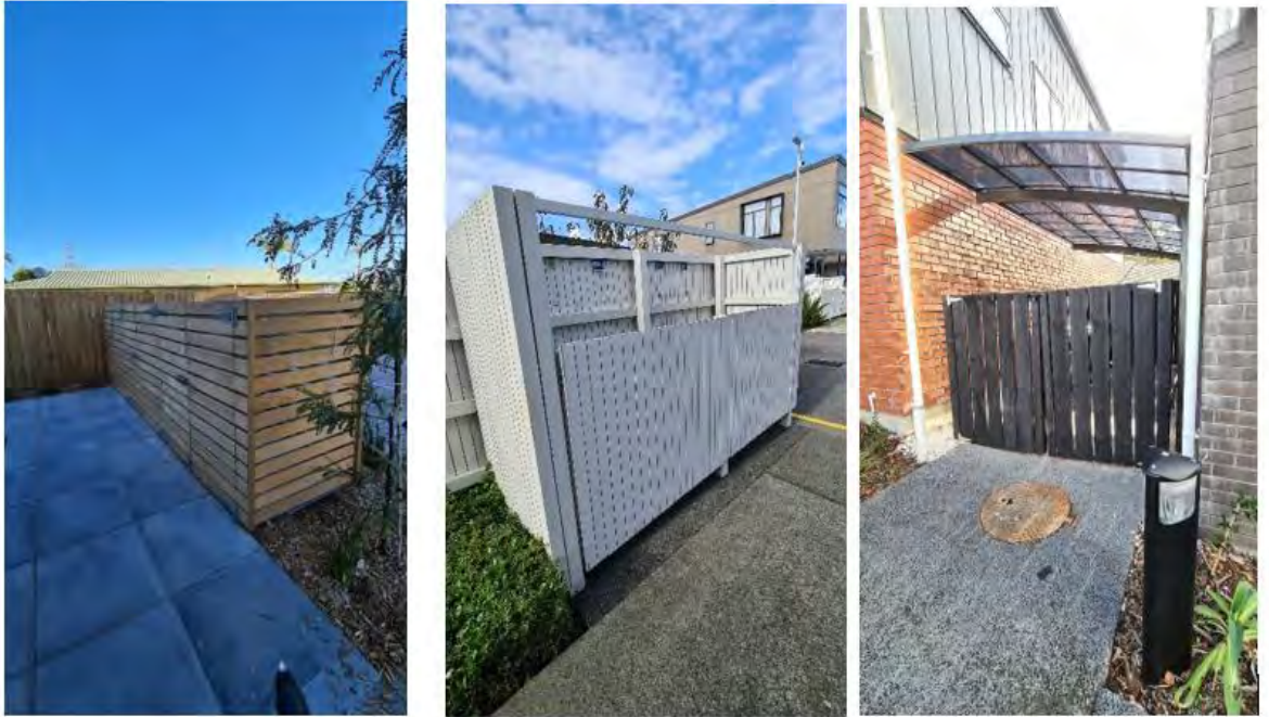
Photos 22, 23 & 24: Communal waste bin enclosures
