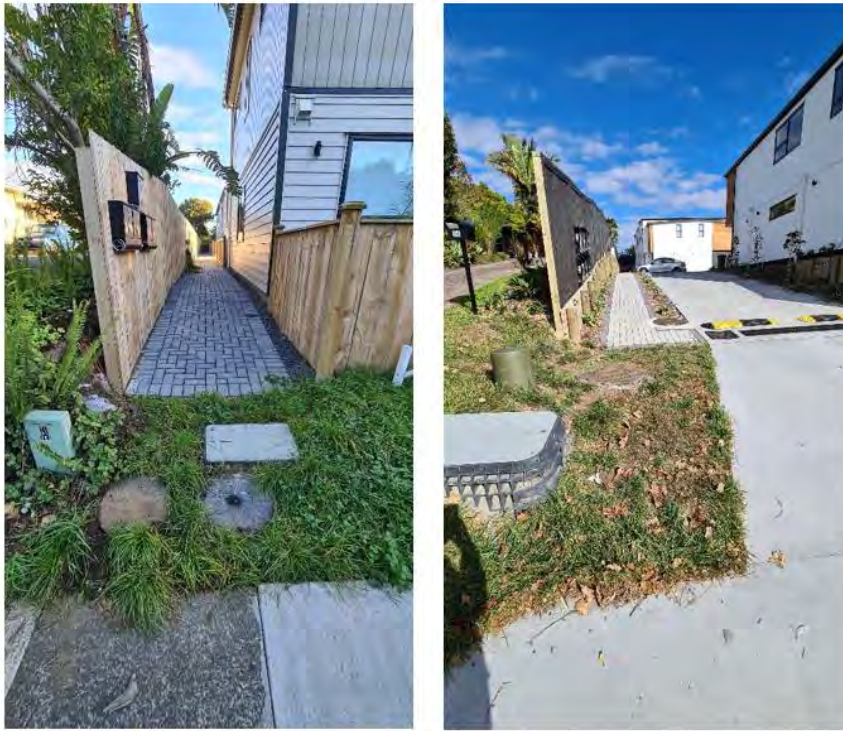
Photos 9 & 10: Pedestrian access routes not connected to public street footpath and utility covers obstructing access
