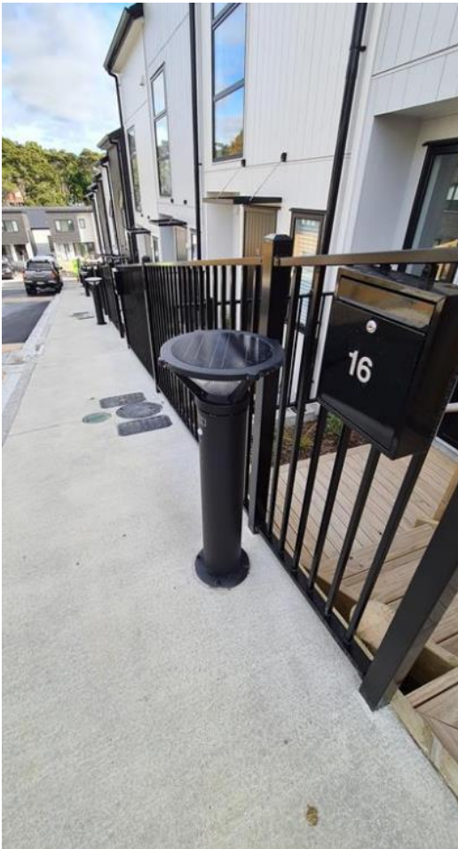
Figure 17: Example of pedestrian access obstruction due to lighting column, 79 College Road, St Johns
