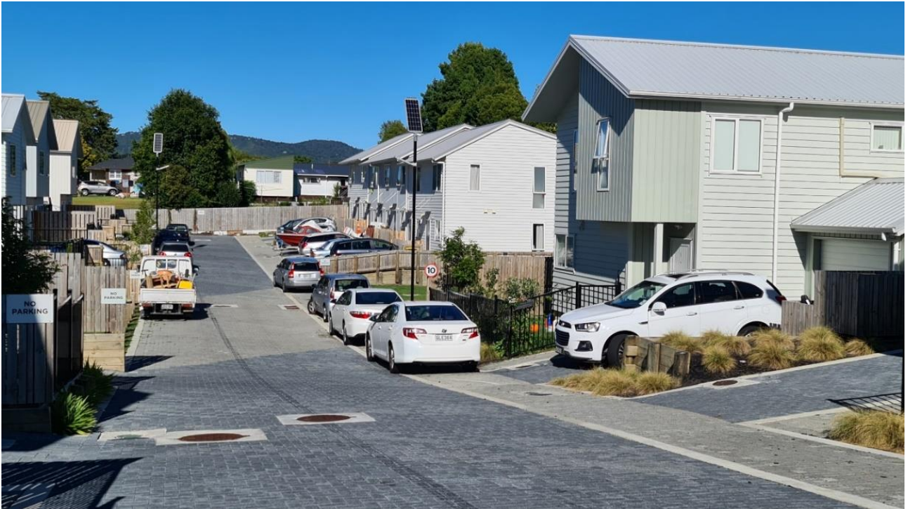
Figure 5: Example of a pedestrian access vertically separated from the carriageway with a curb (Carder Court, Hobsonville)
