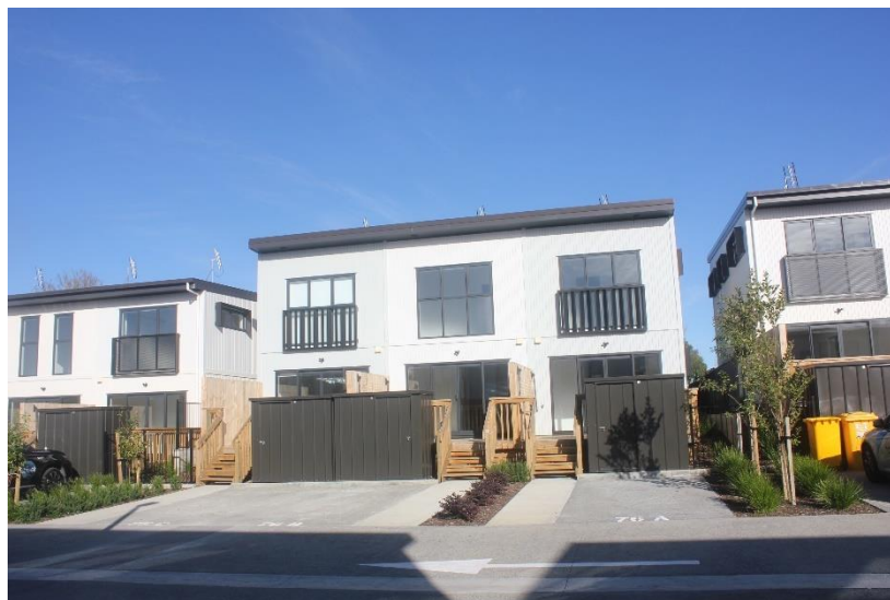
Photo 5: Opaheke Rd, Papakura. Decked outdoor living space with no dedicated space for children to play, with large carpark and shared driveway/manoeuvring space adjacent.
