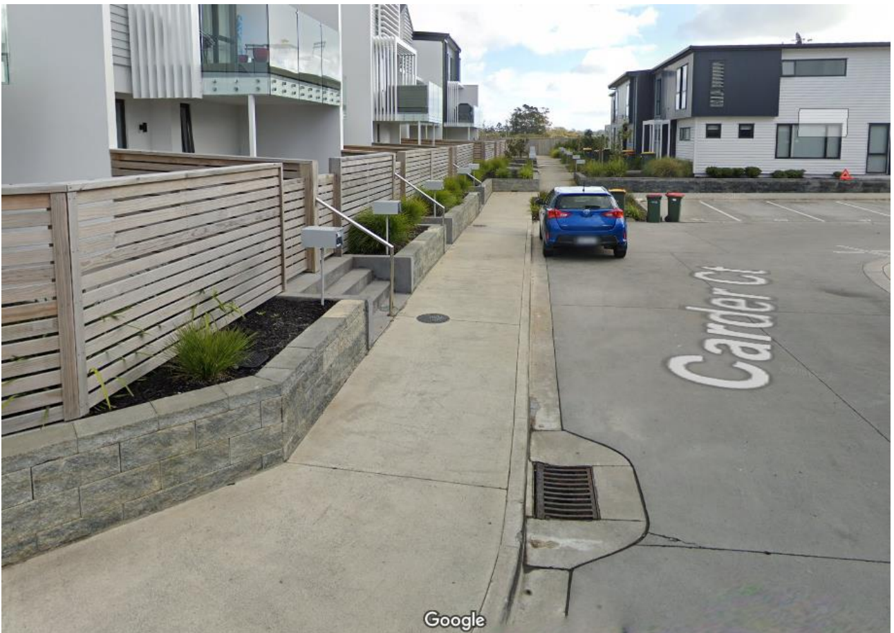
Figure 5: Example of a pedestrian access vertically separated from the carriageway with a curb (Carder Court, Hobsonville)
