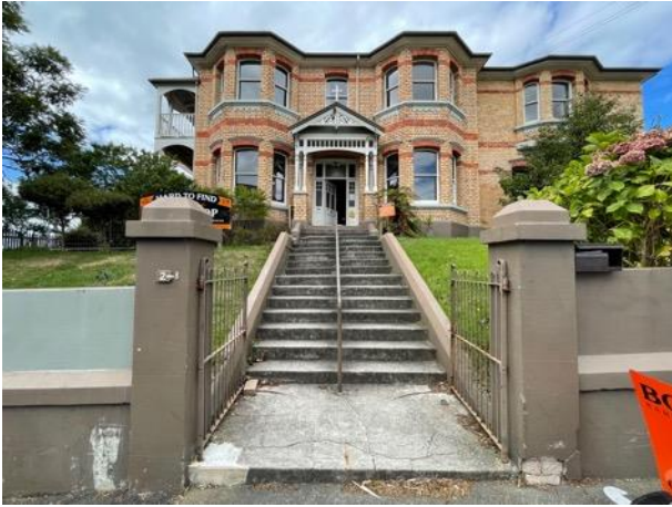
West (front) elevation showing entrance gates and steps.
