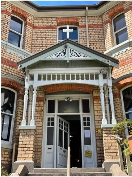
Front entrance porch with decorative timber detailing, front door with top and side lights and double-hung sash windows.
