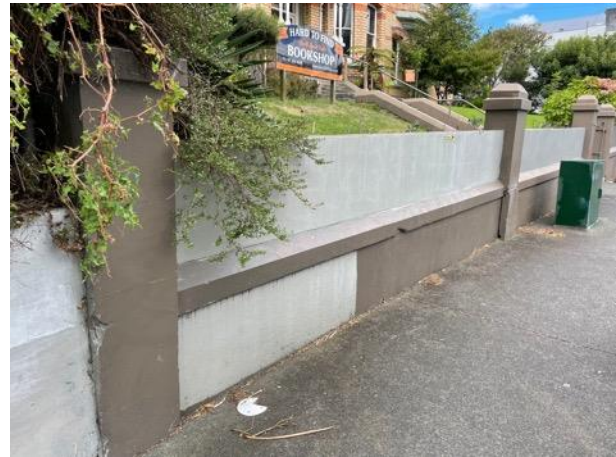
Front boundary plastered brick wall with top panel (replacing earlier railings possibly when the addition was built).
