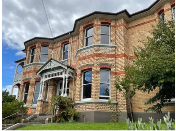
West elevation of the original portion of the convent (1906).
