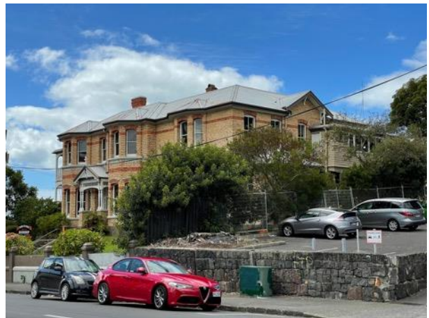
Part south and west elevations, viewed from St Benedicts Street.
