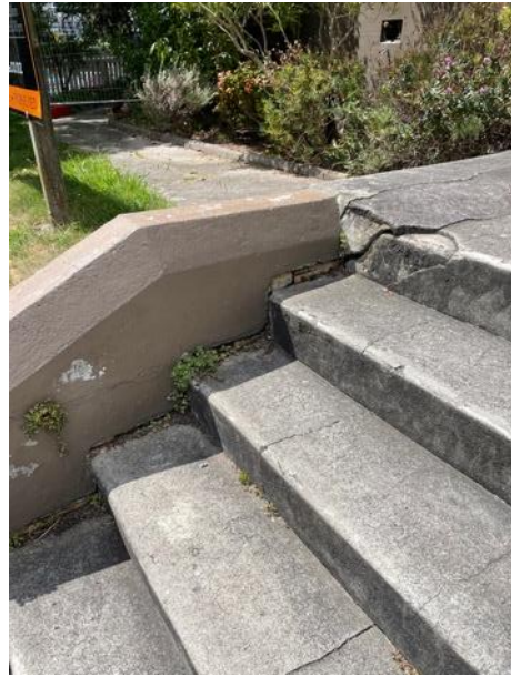
Front entrance steps and plastered brick stringer.
