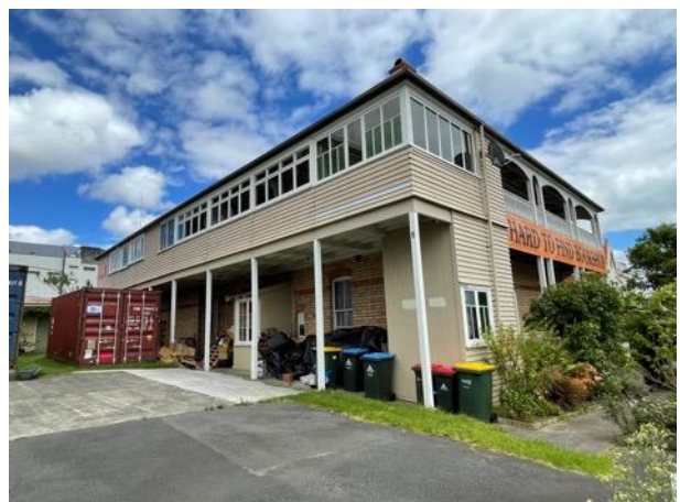
East (rear) elevation showing timber addition, viewed from neighbouring car park.
