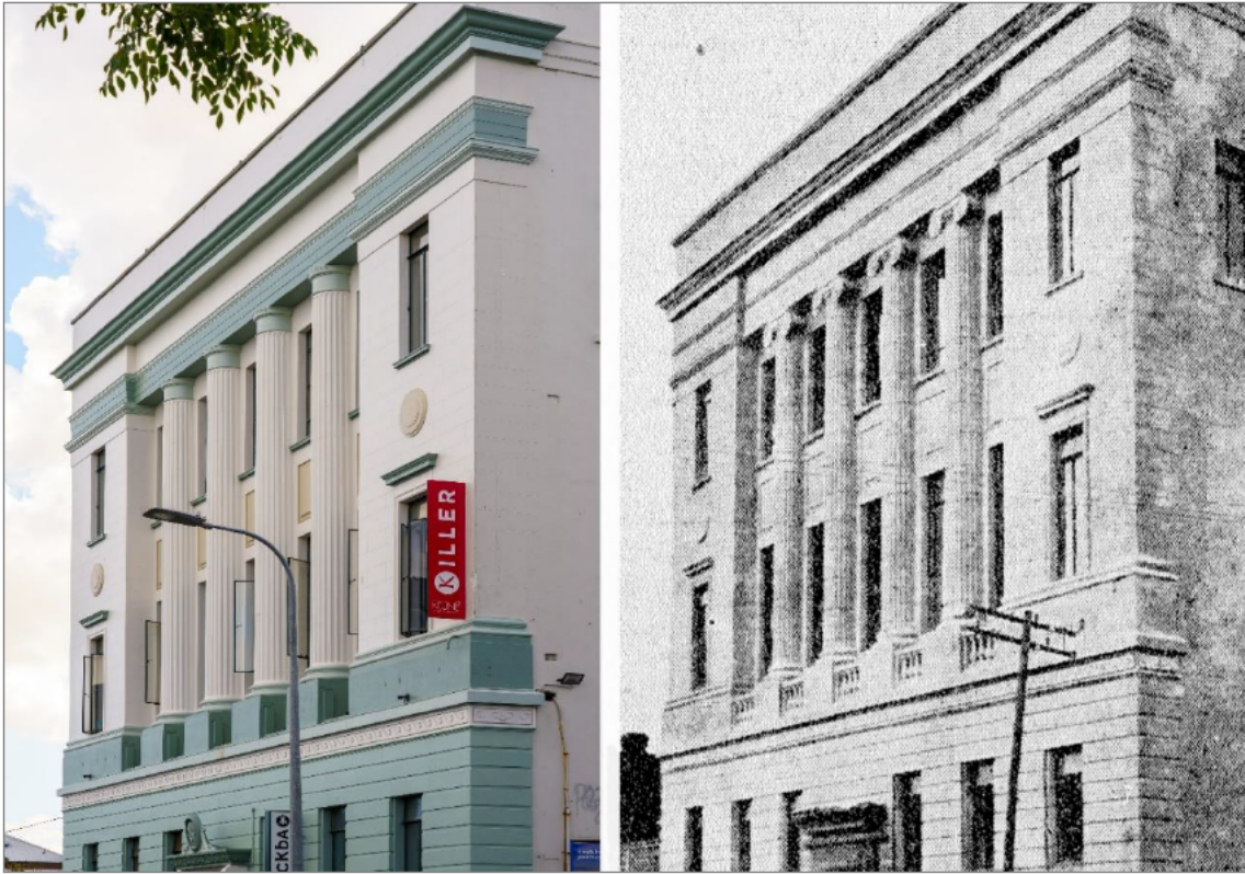
Figure 11: Left: Photograph of the site – Blair Hastings, February 2022. Right: Photograph from June 1930: ‘IMPOSING STRUCTURE IN ST. BENEDICT’S STREET. The new Masonic temple in St. Benedict’s Street is almost complete and in a fortnight’s time should be ready for occupation.’ Sun , 25 th June 1930, p.1. https://paperspast.natlib.govt.nz/newspapers/SUNAK19300625.2.8.1
