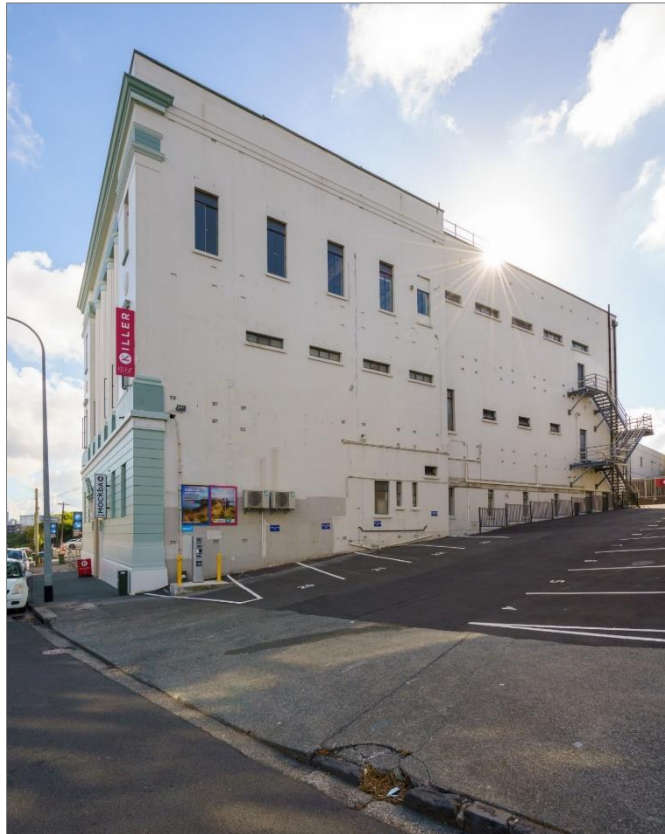
Figure 13: South elevation of the building. Blair Hastings, February 2022.
