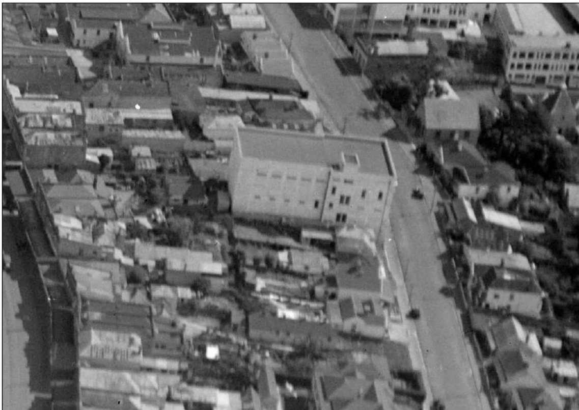
Figure 9: Extract of aerial photograph 1930 - taken from north-east of the site. Shows both the flat roof with which the building was originally built, and also how physically dominant it was, in context with the neighbouring buildings. Whites Aviation Ltd Photographs. Ref: WA-62561-G. Alexander Turnbull Library, Wellington, New Zealand. https://natlib.govt.nz/records/23036926 .
