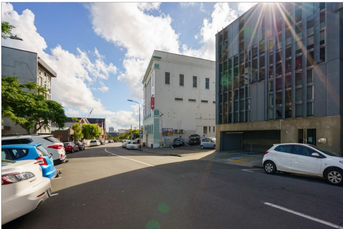
Figure 14: The building – as seen from the south, on St Benedicts Street. Shows the physical dominance the building retains within its local context. Blair Hastings, February 2022.
