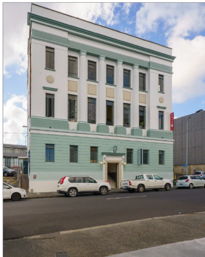
Figure 12: West elevation of the building. Blair Hastings, February 2022.
