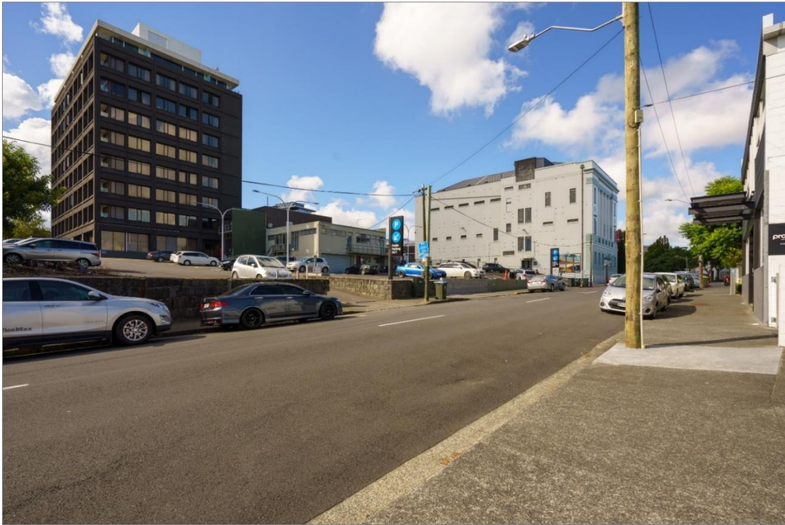
Figure 15: The building – as seen from the north, on St Benedicts Street. Shows the physical dominance the building retains within its local context. Blair Hastings, February 2022.
