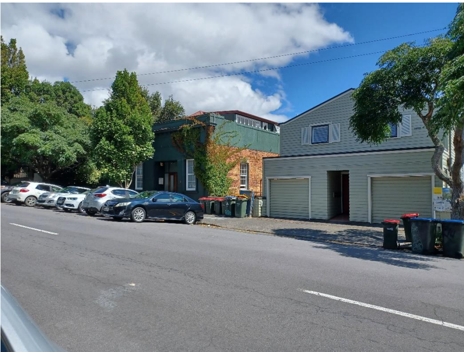
Figure 9: View showing rooftop dormer. (Auckland Council, March 2022)
