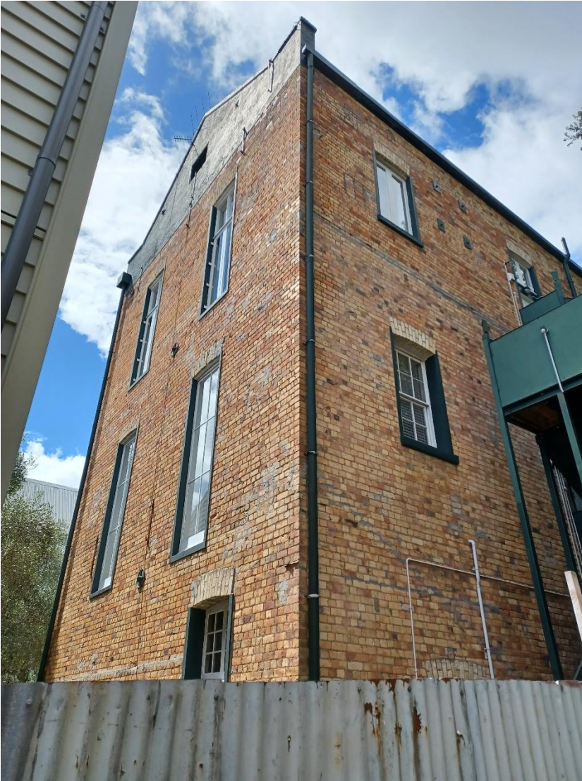
Figure 6: The rear of the building today (Auckland Council, March 2022)
