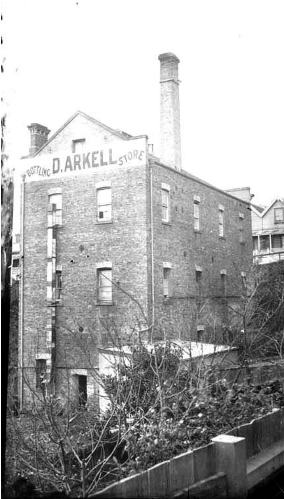
Figure 5: The southern side and the western (rear) view of the bottling store in the late 19 th or early 20 th century, showing access from Randolph Street. (Auckland Libraries Heritage Collections 4 -RIC97)
