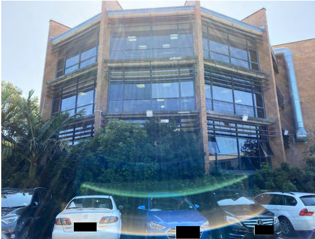
The southern and western elevation of the building.
