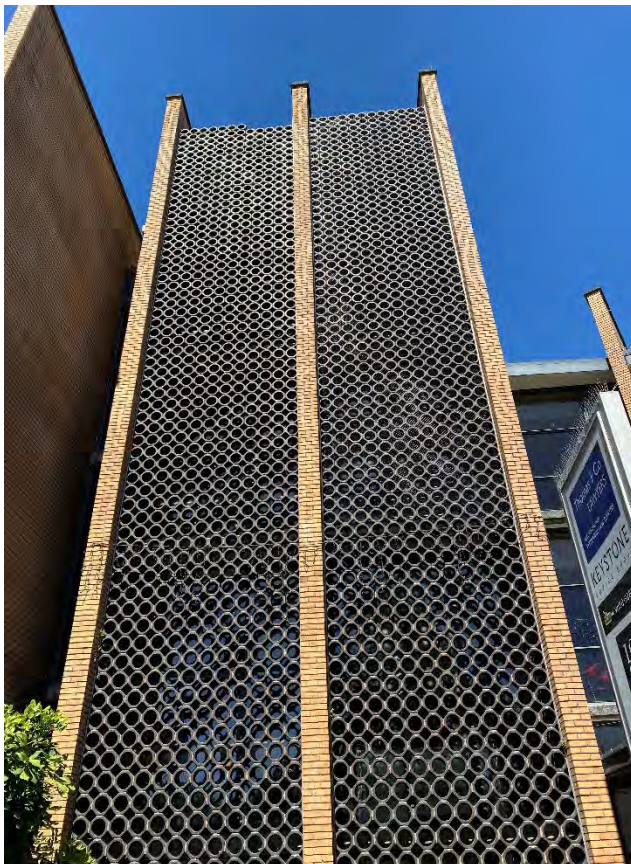
The ceramic pipes screening the stairwell and lift chamber.
