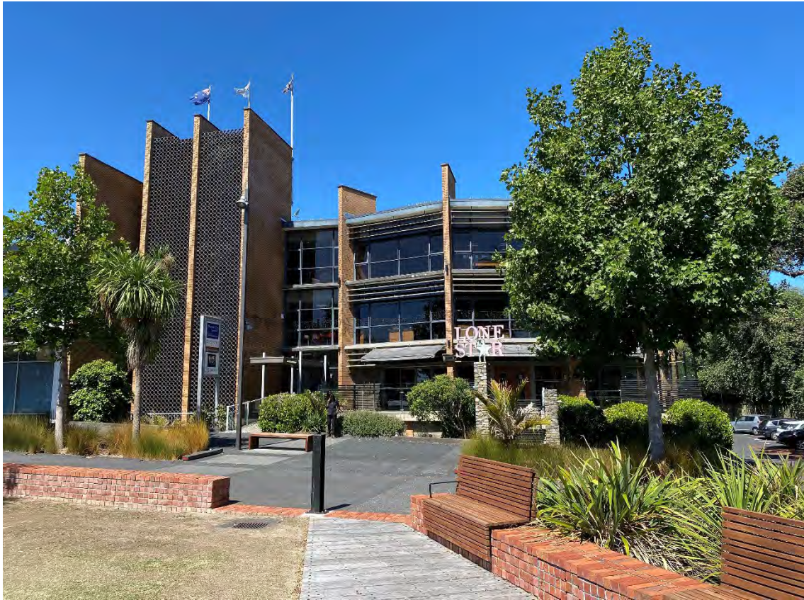
The northern elevation of the building.
