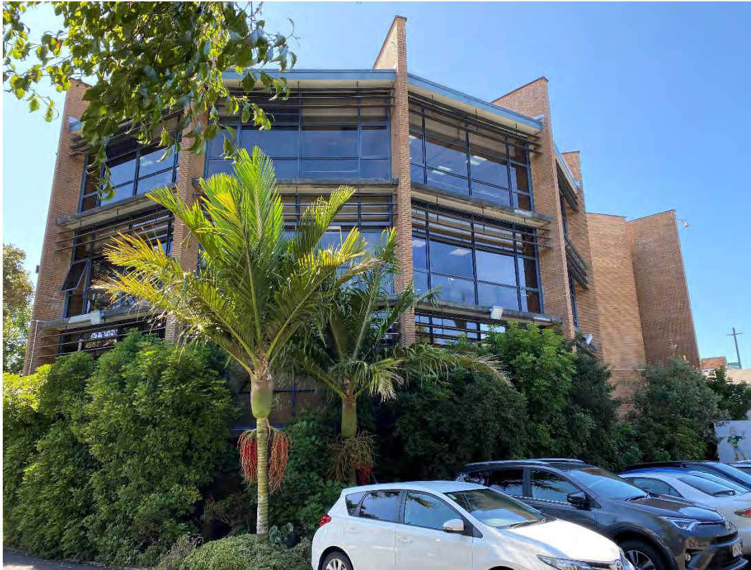
The western elevation of the building.
