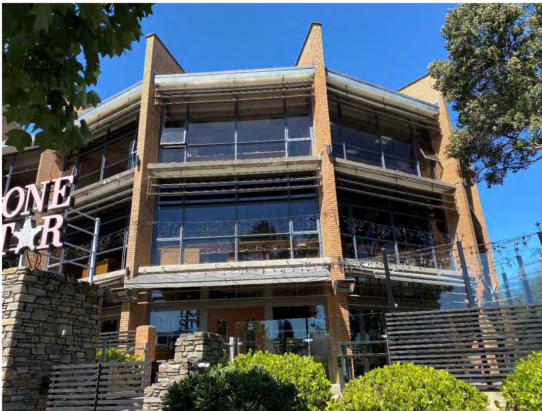
The front (northern) elevation of the building.
