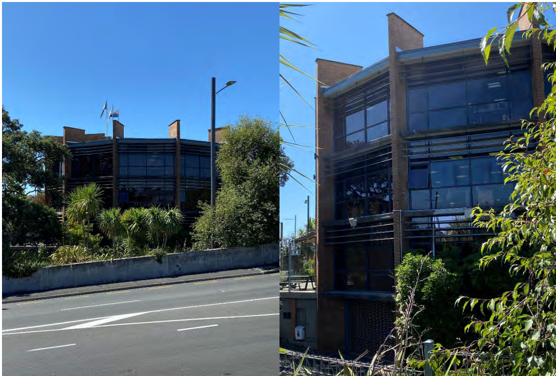
The western elevation of the building.
